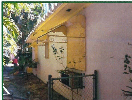
Figure 15: 229 Ridgewood Road, Side (East) Façade, May 2016
