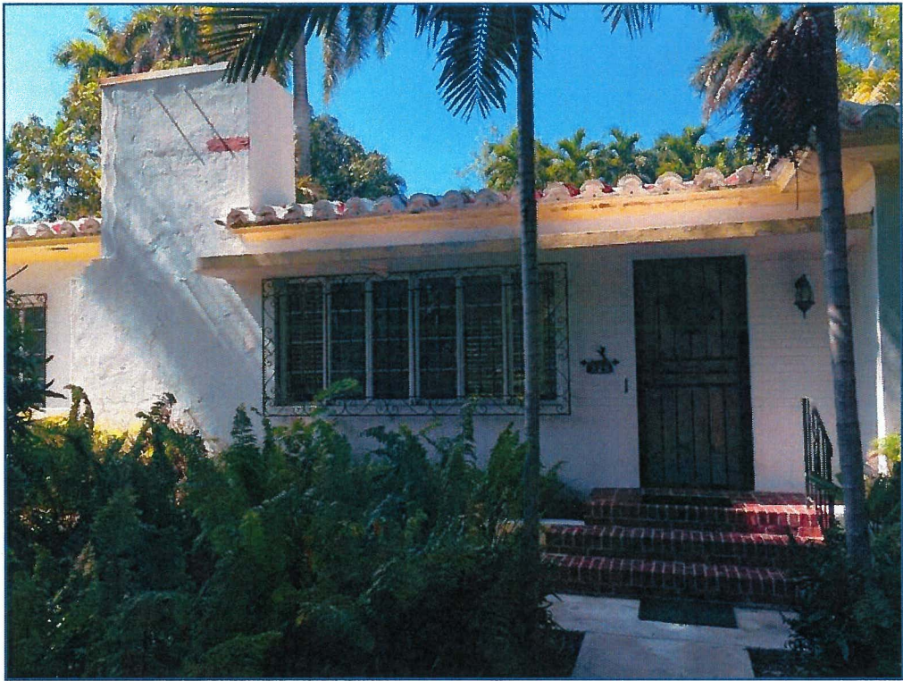
Low-pitched hipped roofs with white two-piece barrel tile
