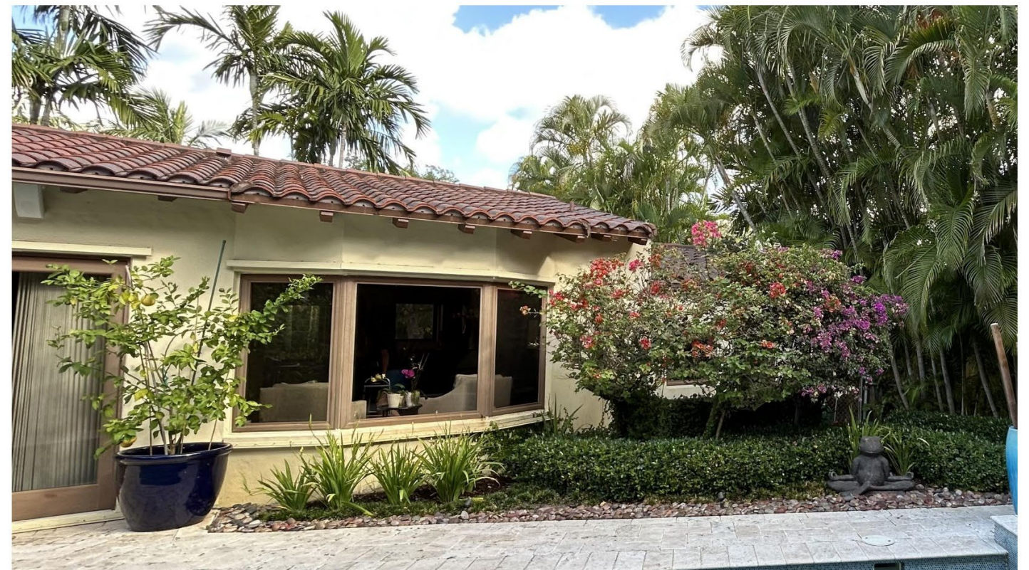
View of Rear
