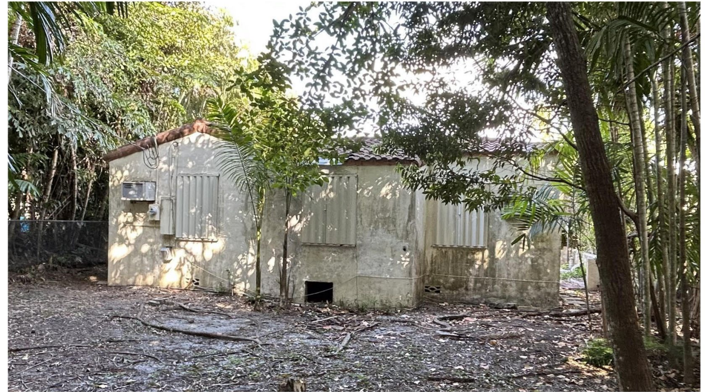
View of Rear
