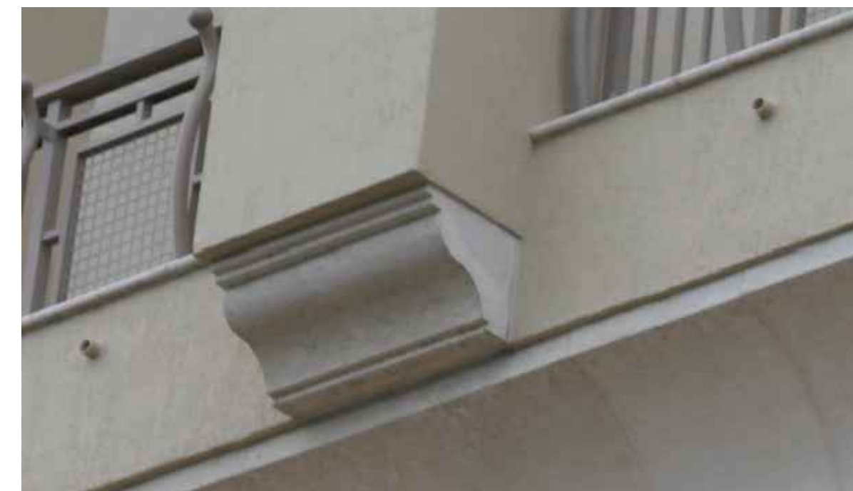
8 PRECAST CONCRETE BRACKETS GABLES PONCE
