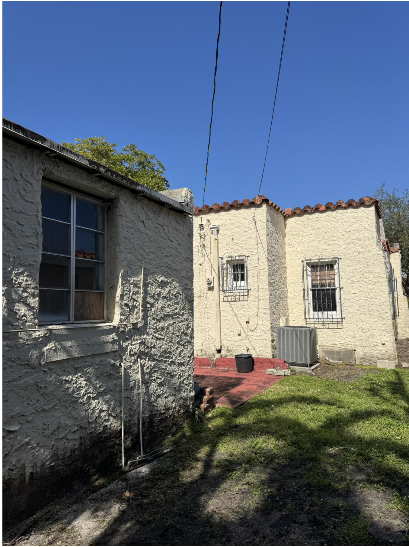
SIDE YARD VIEW SHOWING THE BACK OF THE EXISTING DETACHED GARAGE AND MAIN BUILDING
