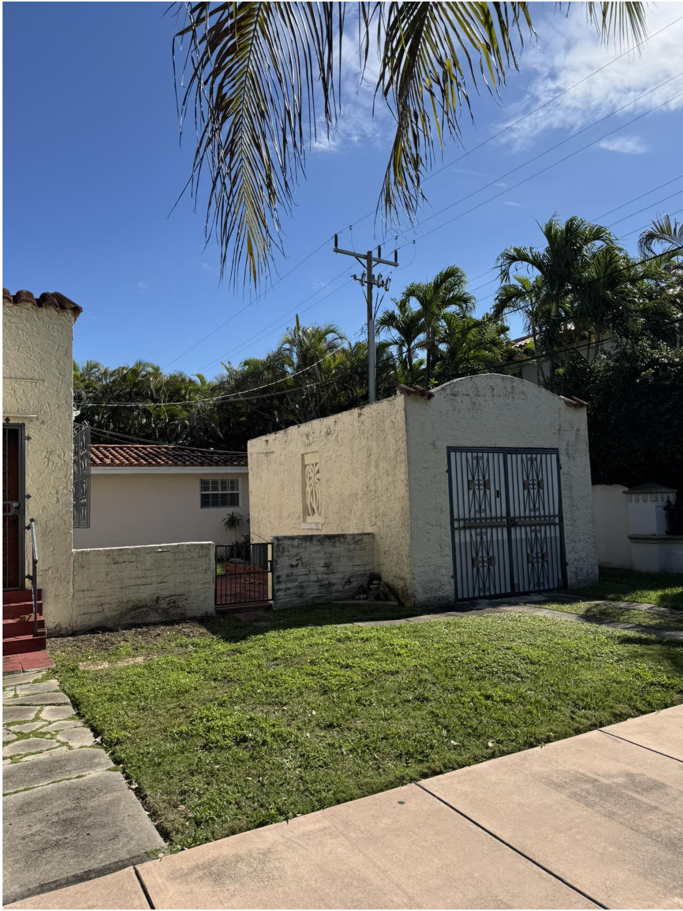
VIEW OF EXISTING DETACHED GARAGE BUILDING FROM HERNANDO STREET
