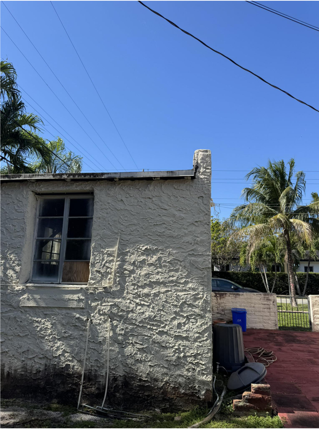
EXISTING DETACHED GARAGE BUILDING
