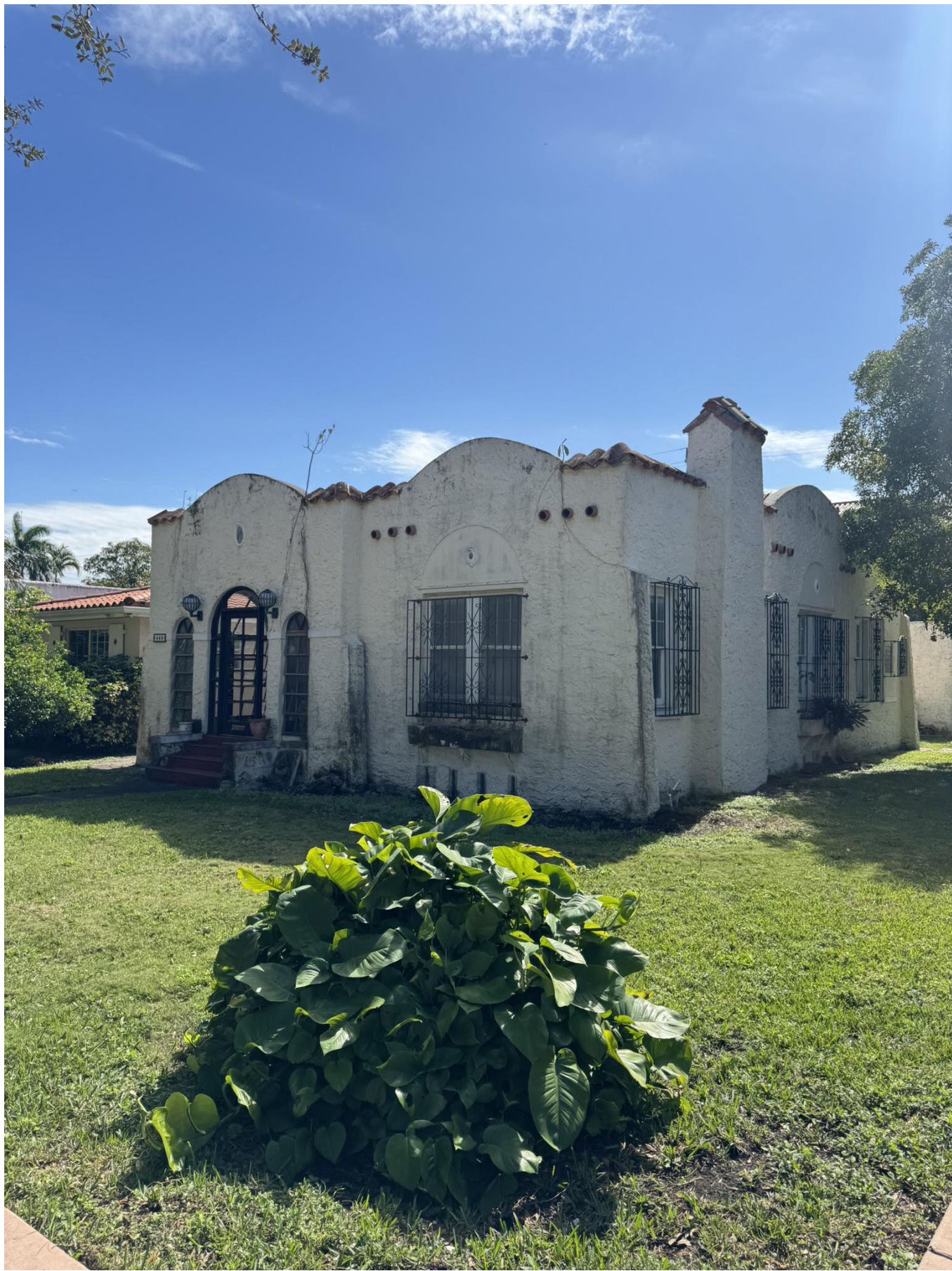
VIEW FROM THE CORNER OF ARAGON AVENUE & HERNANDO STREET
