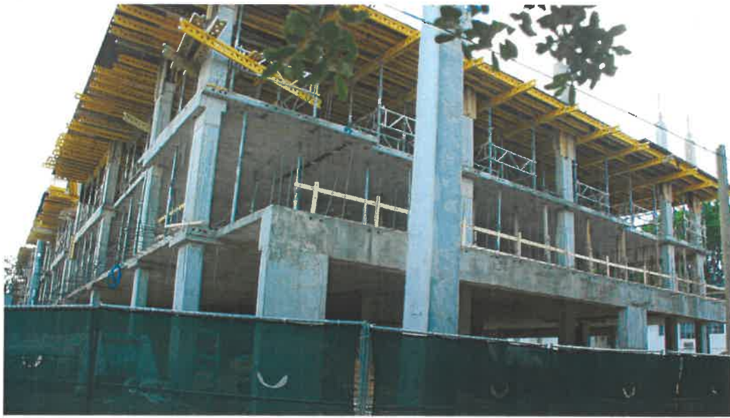
Valencia Avenue - Adjacent Property
