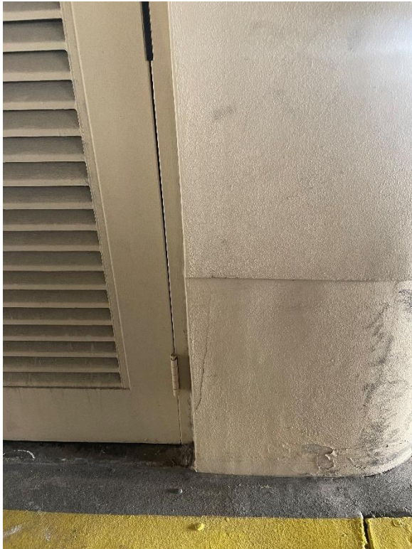
Photo 25: Typical louvered hollow metal door in the garage.
