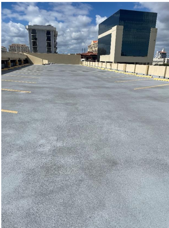
Photo 19: Existing waterproofing of the top garage deck.
