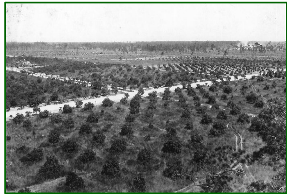
Figure 2: Streets in Coral Gables under Construction, July 22, 1922
