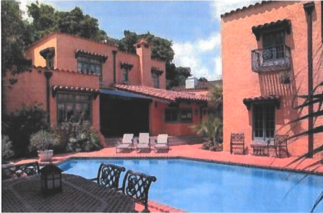
Location of expansion and renovation. Lower sloped roof to be removed and replaced with taller flat roof with covered terrace and renovated pool
