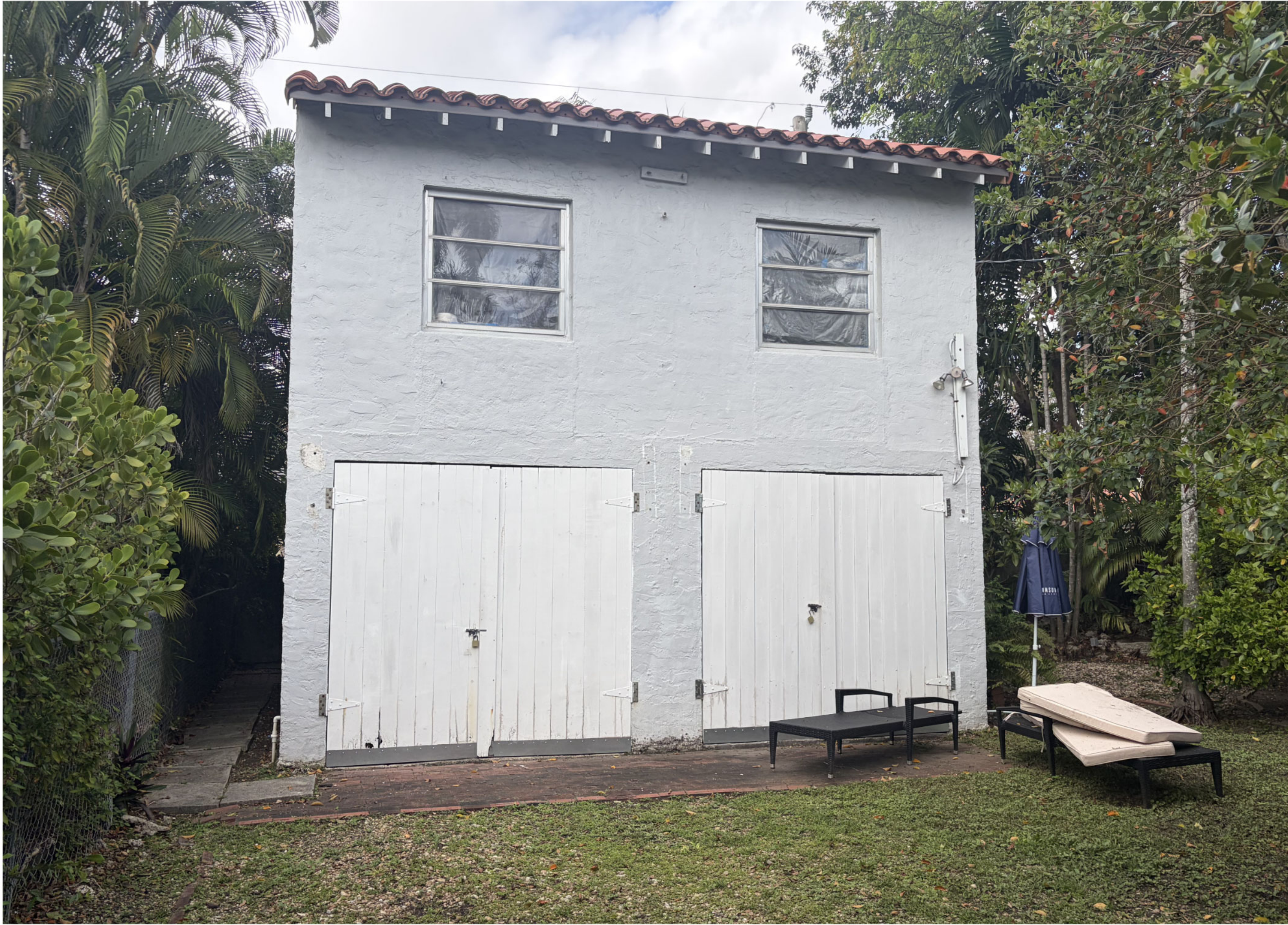
Existing carriage house
