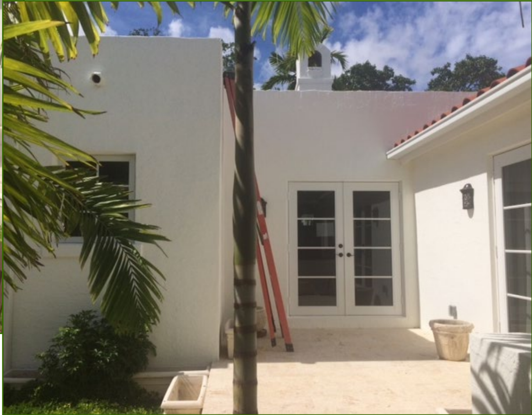
South (Rear) Façade – After
