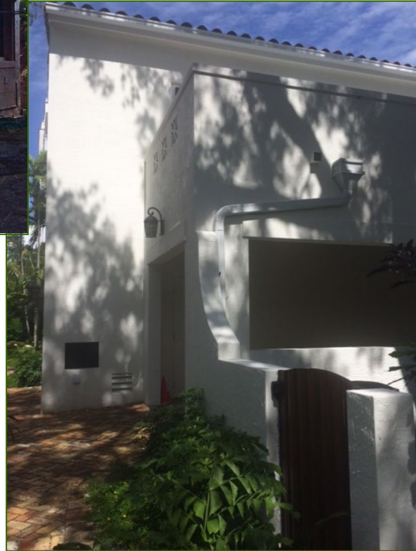
West Façade – Before & After
