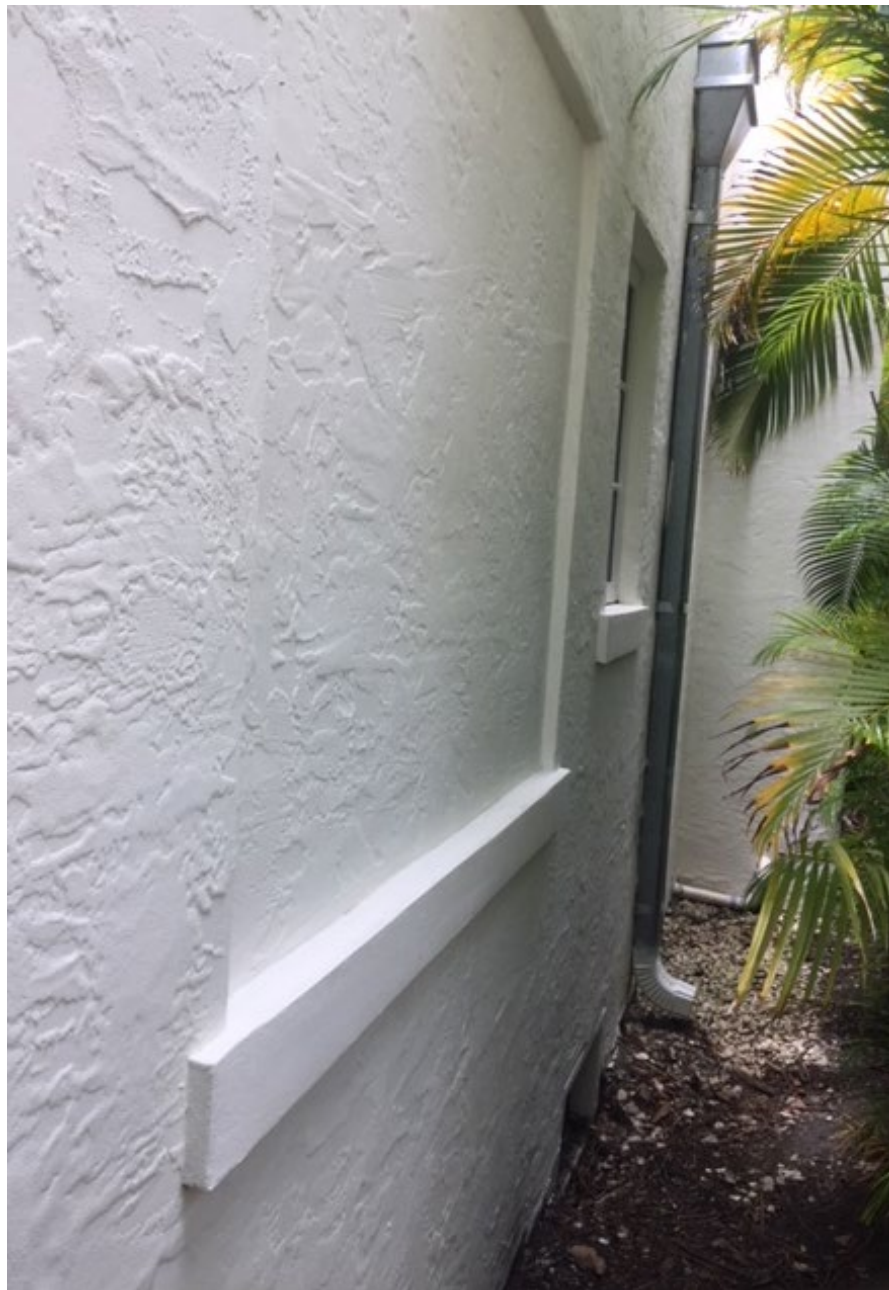
East Façade – Window “Memory” After
