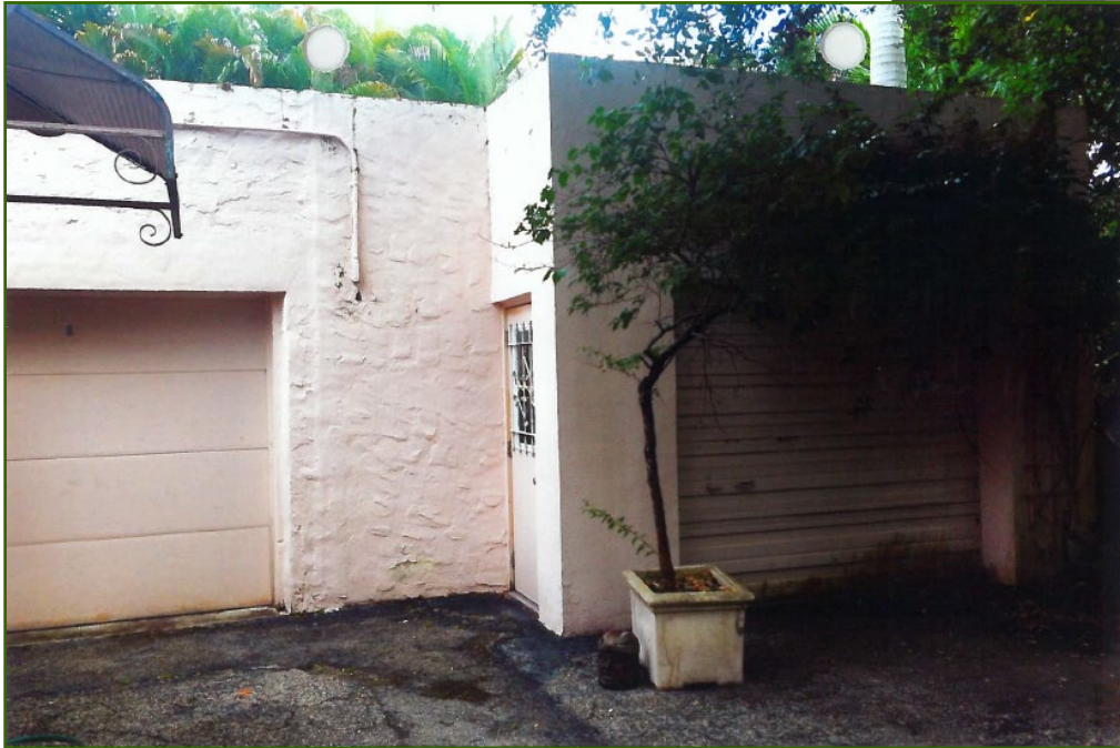
North (Front) Façade Garage – Before & After
