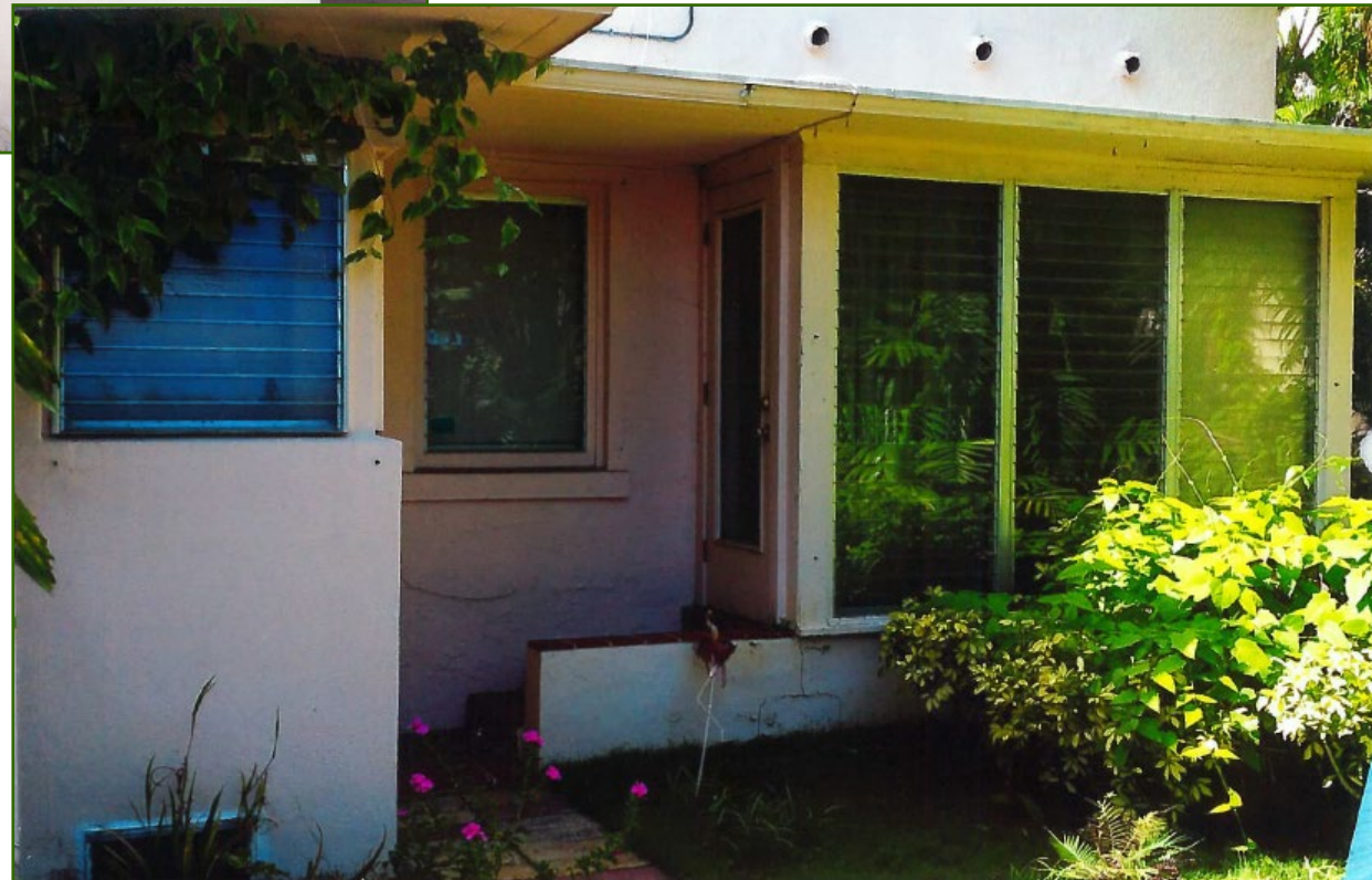
South (Rear) Façade – Before
