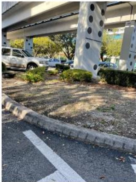
Figure 18 Lack of landscaping in parking curb.
