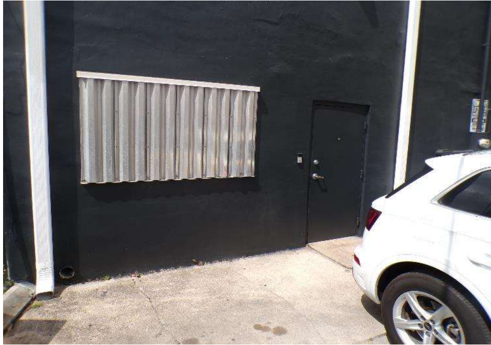
A steel door in the east exterior wall
