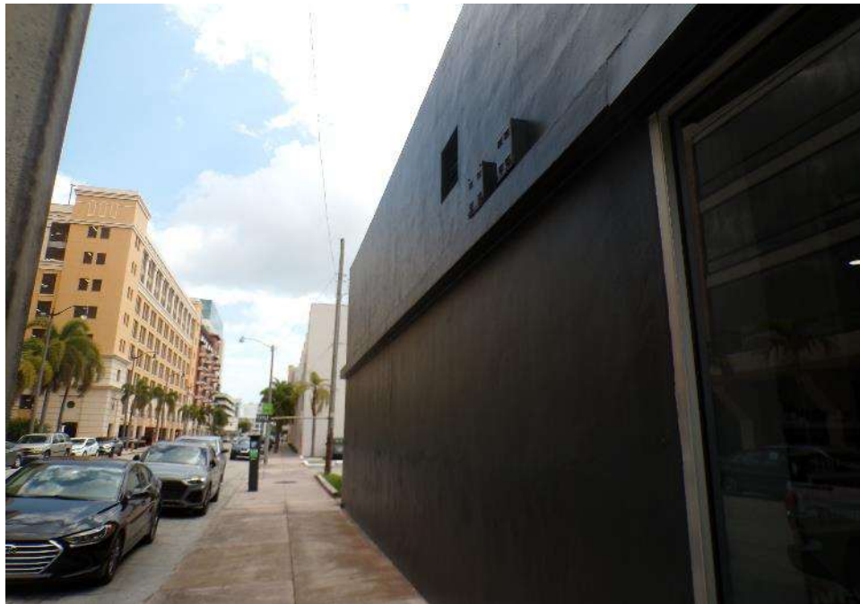
Partial north-facing elevation of the building
