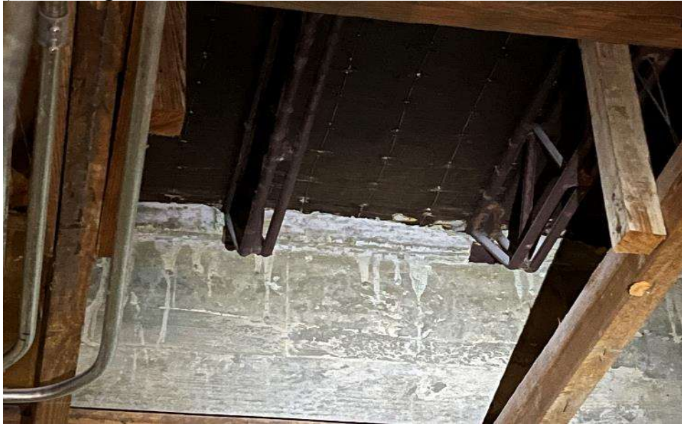
Typical CIP concrete tie beams along the building's exterior walls
