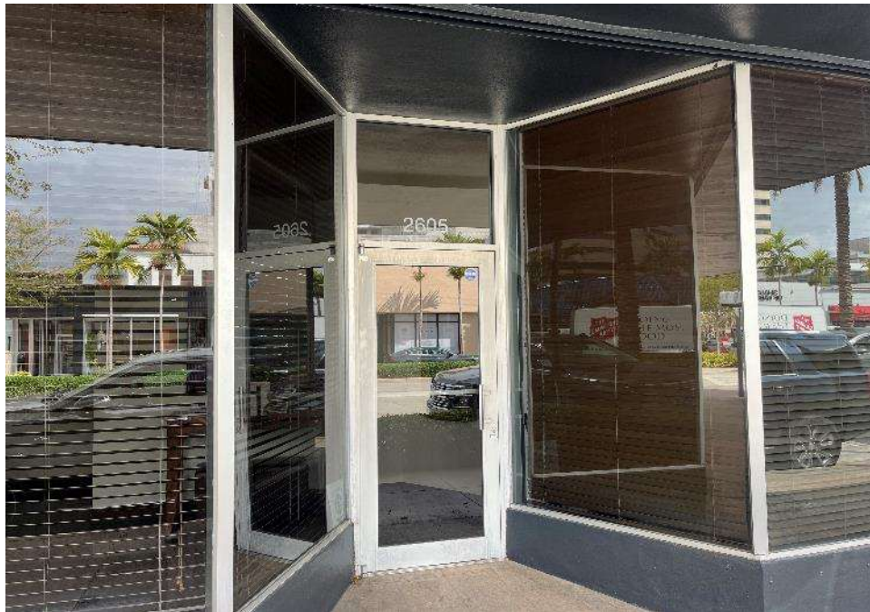
Typical aluminum-framed glass doors along the building's storefront
