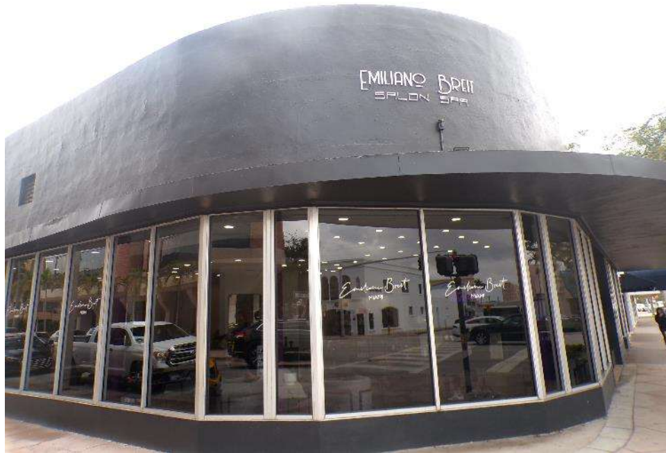
Northwest corner of the building
