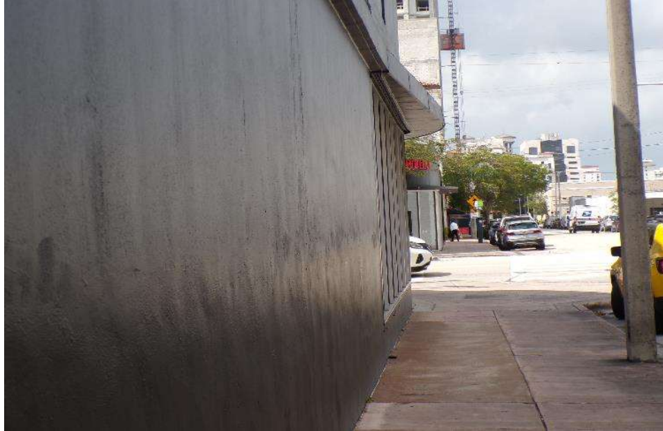
Typical painted stucco along the building's facade
