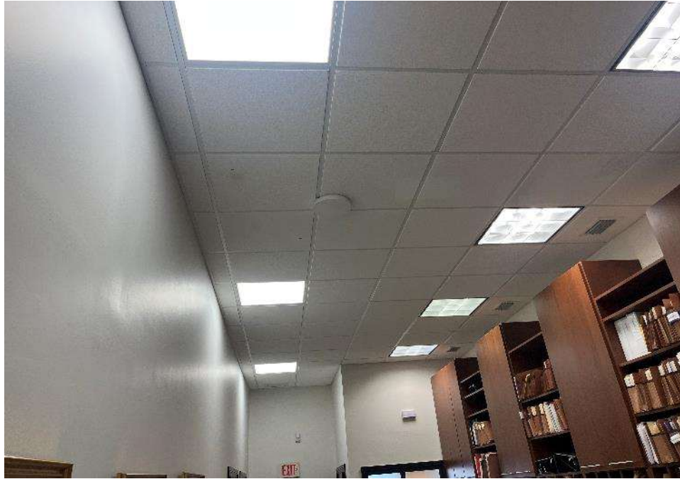
Typical interior finishes in Unit 2605
