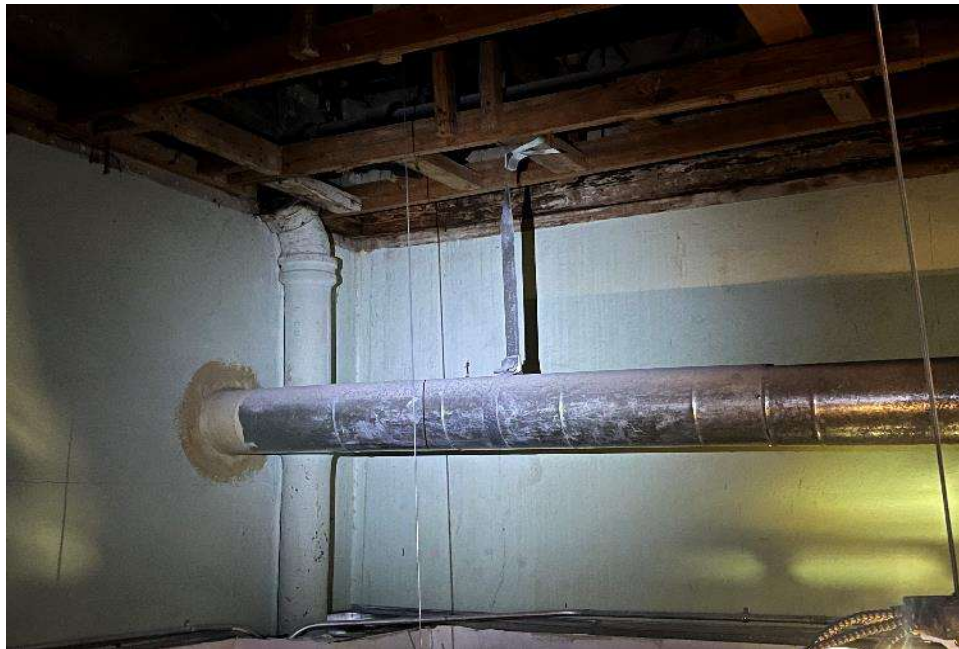
Typical plaster along the interior finish of the CMU exterior walls
