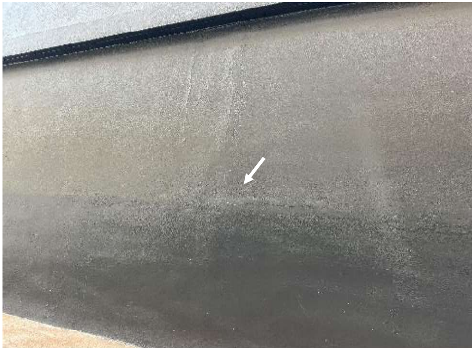
Previous stucco repairs along the building facade
