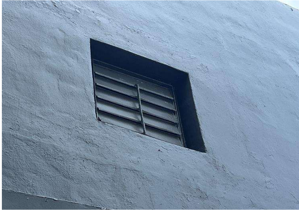
Typical metal awning windows along the north elevation of the building
