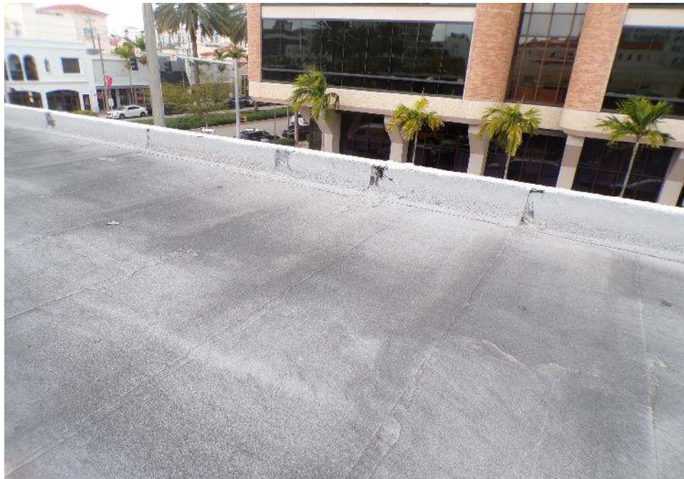
Typical low CMU parapet of the building
