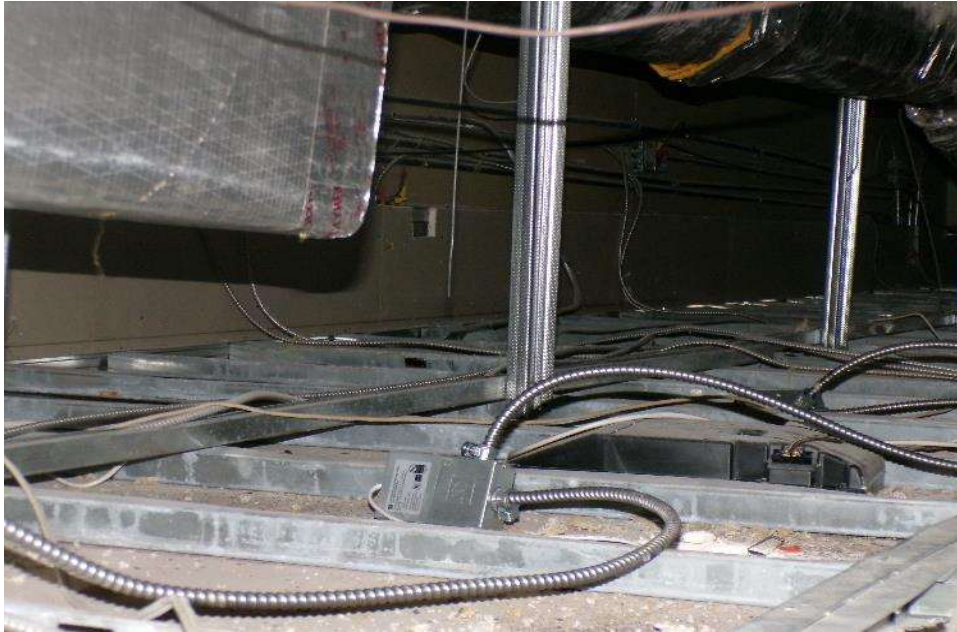
Typical drywall along the partition walls
