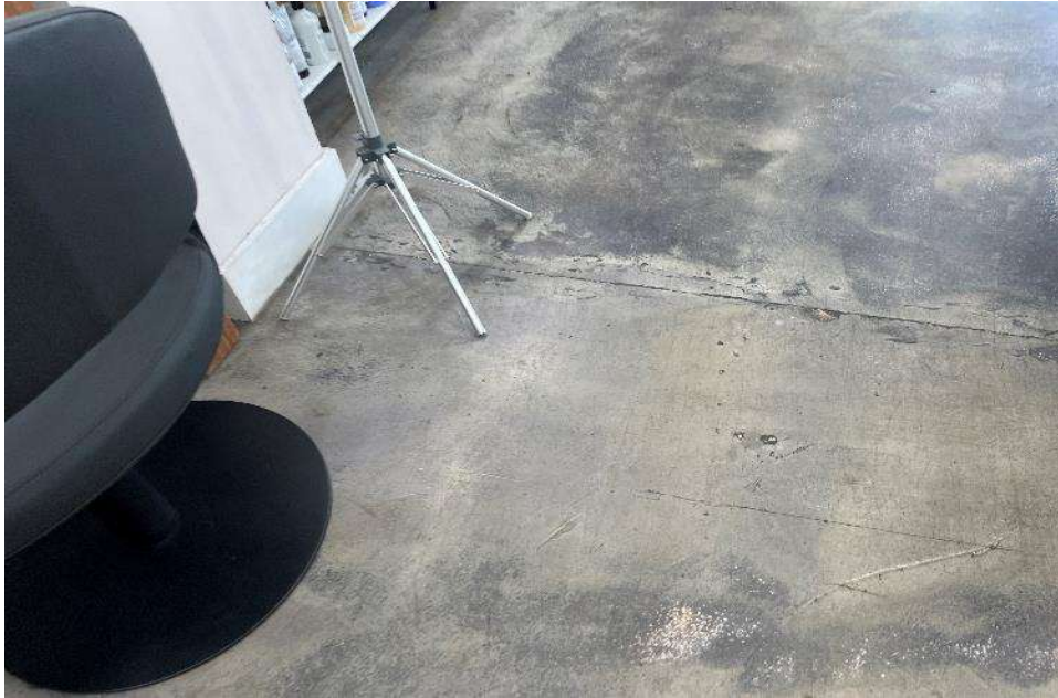
Typical concrete SOG of the building
