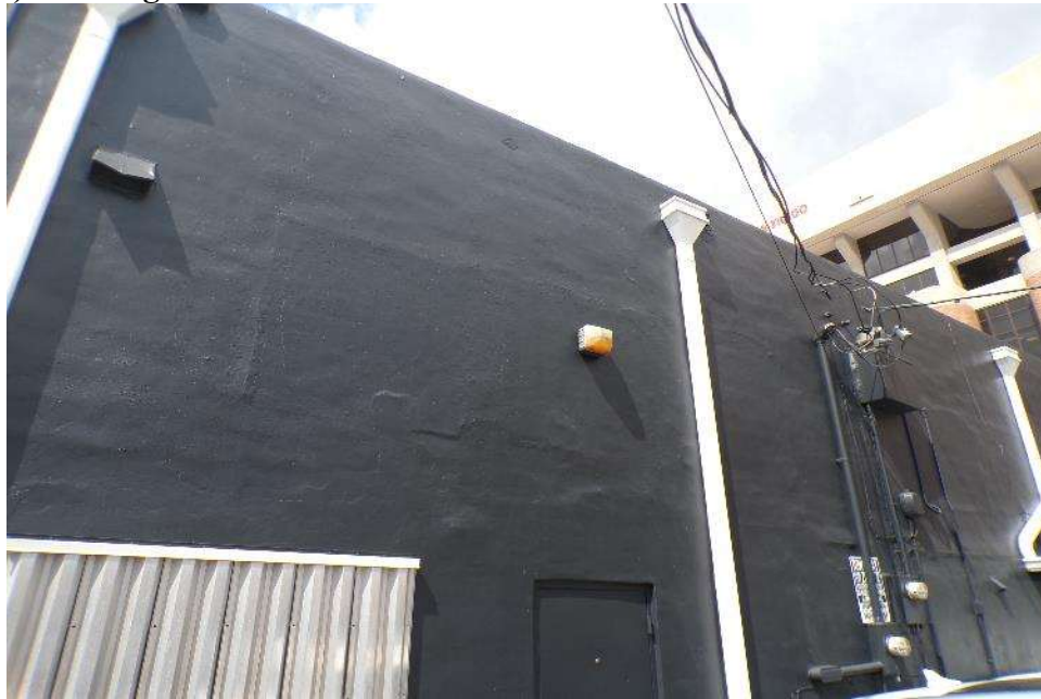
Typical exterior CMU walls
