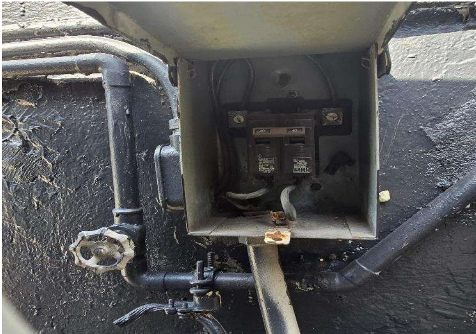
27.4 A C Disconnect switch - PROVIDE GROUND WIRE
