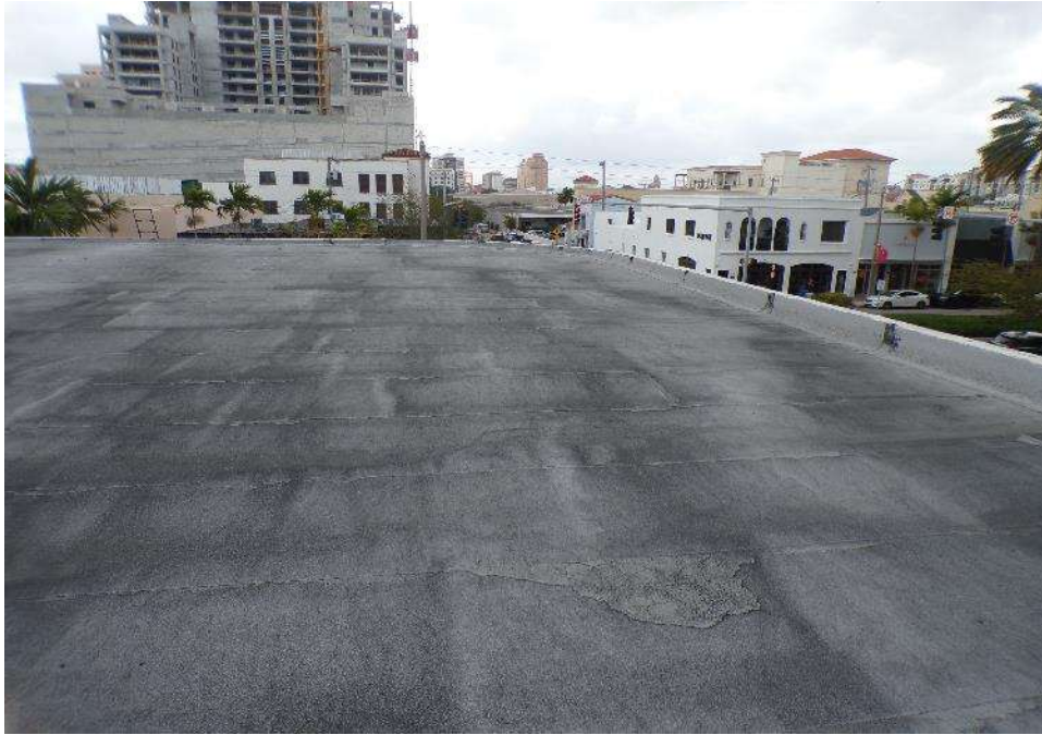
Modified bitumen membrane looking east on the roof
