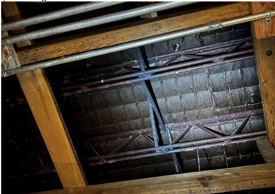
Typical open web roof trusses of the building
