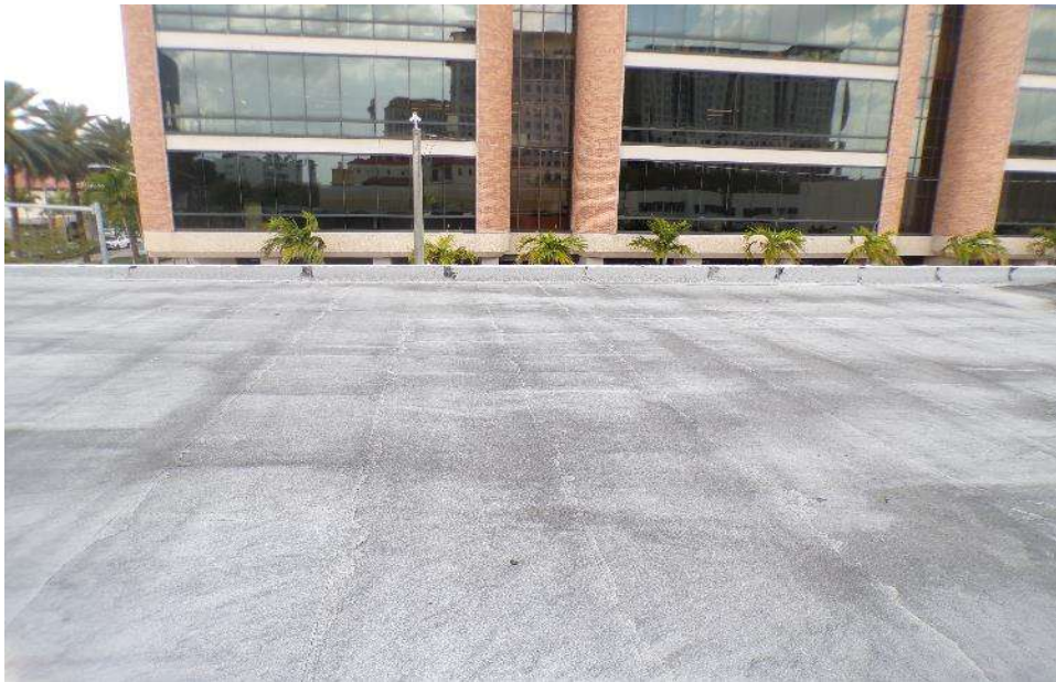
Modified bitumen membrane looking north on the roof
