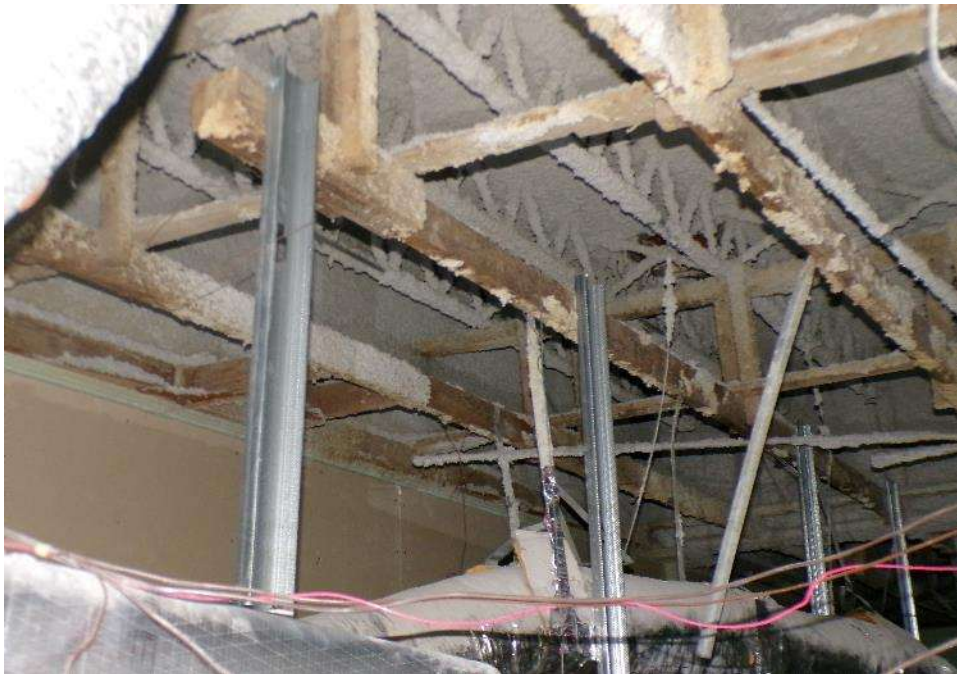
Applied fireproofing along to the roof structures in Unit 2603
