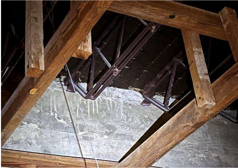
Typical connections of the roof trusses to the exterior CMU walls
