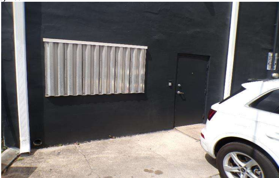
Windows in the west exterior wall are covered with metal shutters
