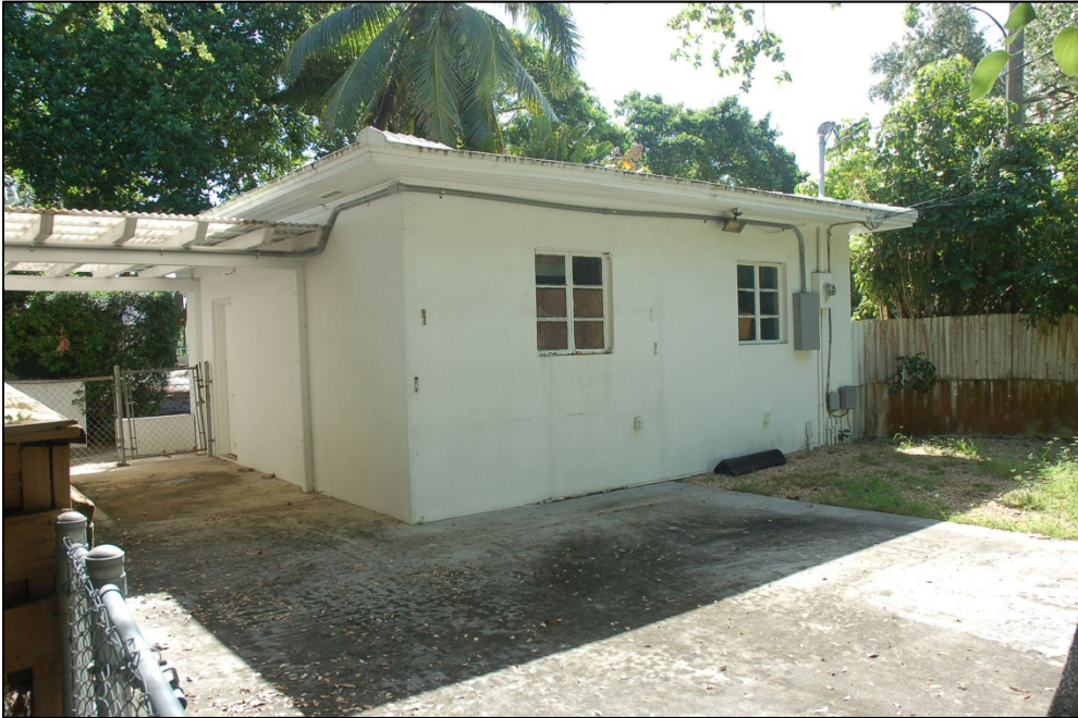
View of rear of detached garage.
