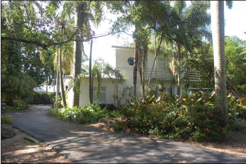
View of main residence looking southerly.
