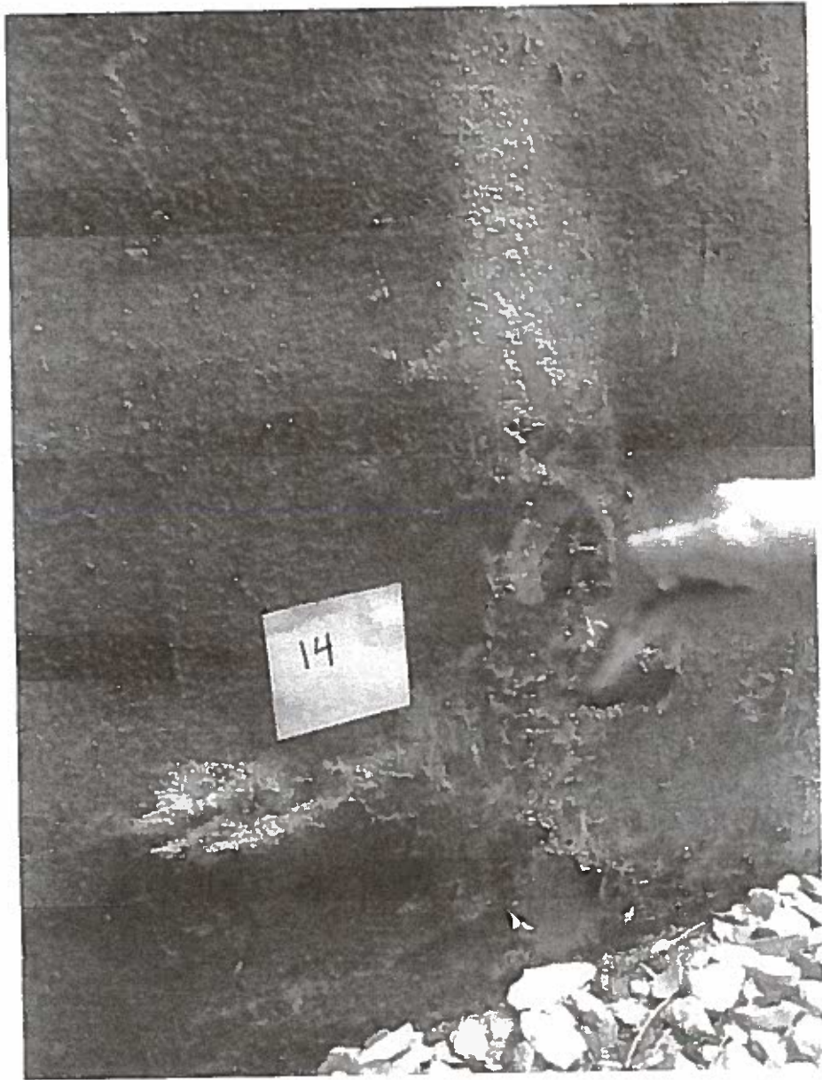
Exterior Wall: Picture 7
