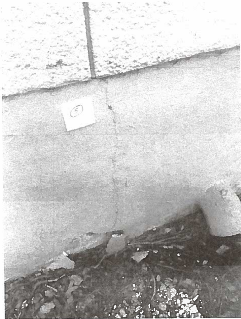
Exterior Wall: Picture 5
