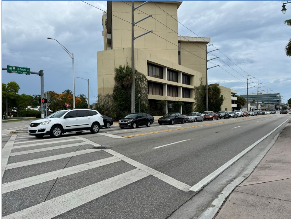
Photo 3 – Westbound traffic queues on SR 90/SW 8 th Street at Ponce De Leon Boulevard reaching Galiano Street
