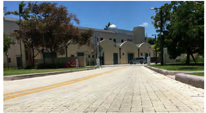
Physics Controlled Access Service Road
