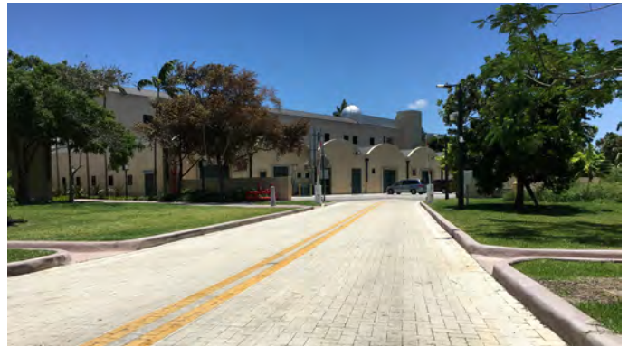
Controlled Access Service Road behind Physics Building
