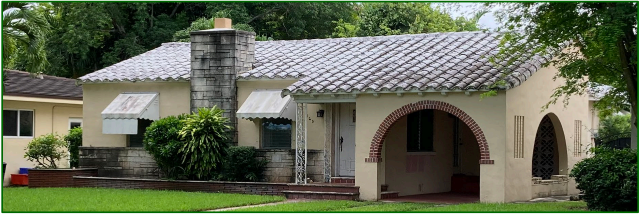
Figure 17: Front (North) Façade, 2024
