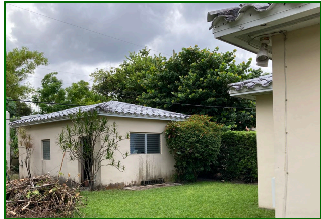
Figure 23: Original Detached Garage, Now a Storage Building, 2024
