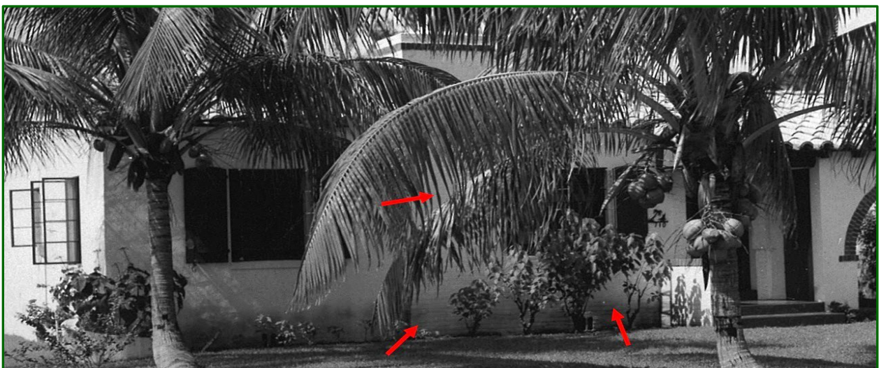
Figure 18: Front (North) Façade, c.1940s Note: Spiral Planter at NE corner Red Arrows: slump brick
