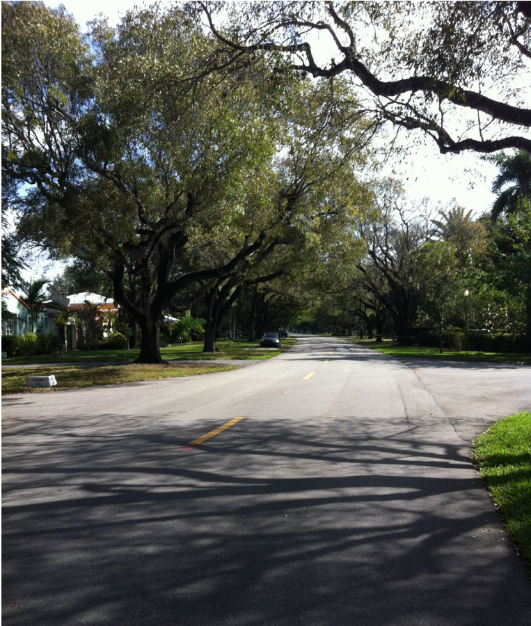
4. AMPLE PAVEMENT Existing lanes are wide along this stretch of University Drive and could use a road diet.
