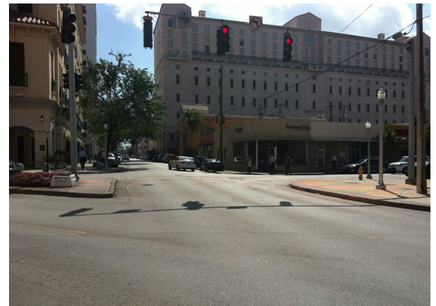
5. MESSY INTERSECTION. The intersection of Galiano and Giralda is confusing for pedestrians and cyclists. Adding crosswalks and expanding pedestrian islands can fix this problem.
