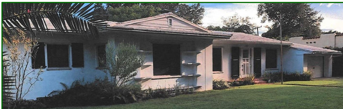
Figures 1: 1208 Asturia Avenue, Front (North) Elevation -- c.1940 [top]; 2019 [bottom]
