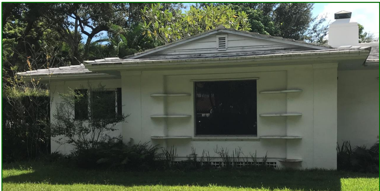
Figures 18: Front Façade, Central Projecting Bay Note: Sculptural shelving, Inset for window, Corner pilaster, Wood siding in gable end
