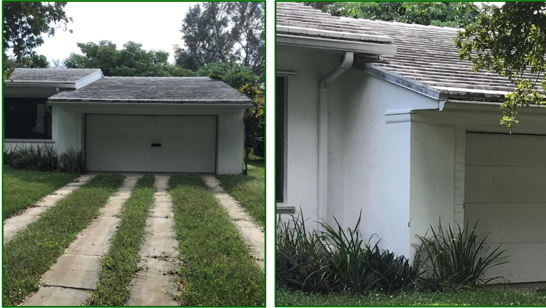
Figures 21: Garage Bay, 2019 Note: Corner pilaster and Masonry block framing opening
