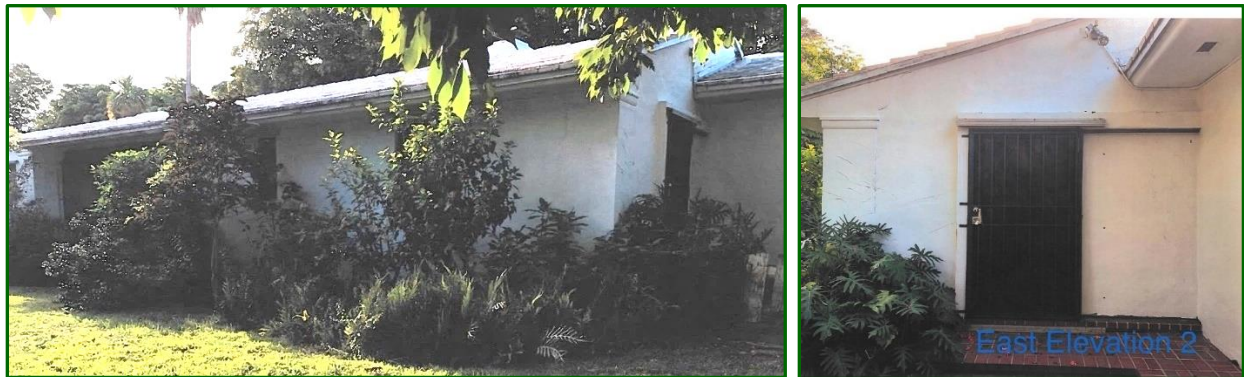
Figures 23: 1208 Asturia Avenue, 2019, photos provided by applicant South elevation looking northwest [left] East elevation (bedroom #3) rear of home [right]
