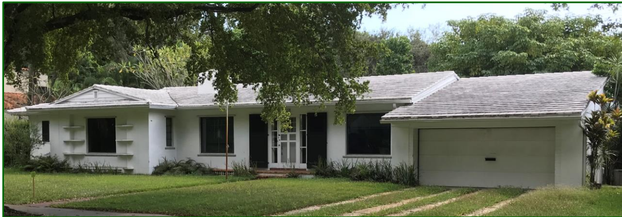
Figures 16: 1208 Asturia Avenue, Front (North) Facade, looking southeast, 2019
