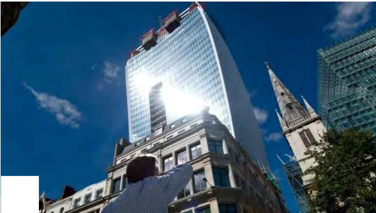
The BBC's Andrew Verity surveys the damage caused by the skyscraper
