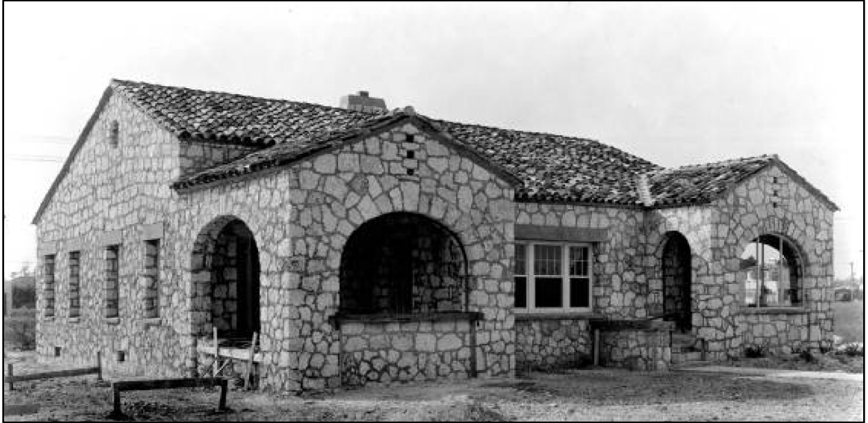
Figure 1: November 15, 1923 Fishbaugh photo, Under Construction
