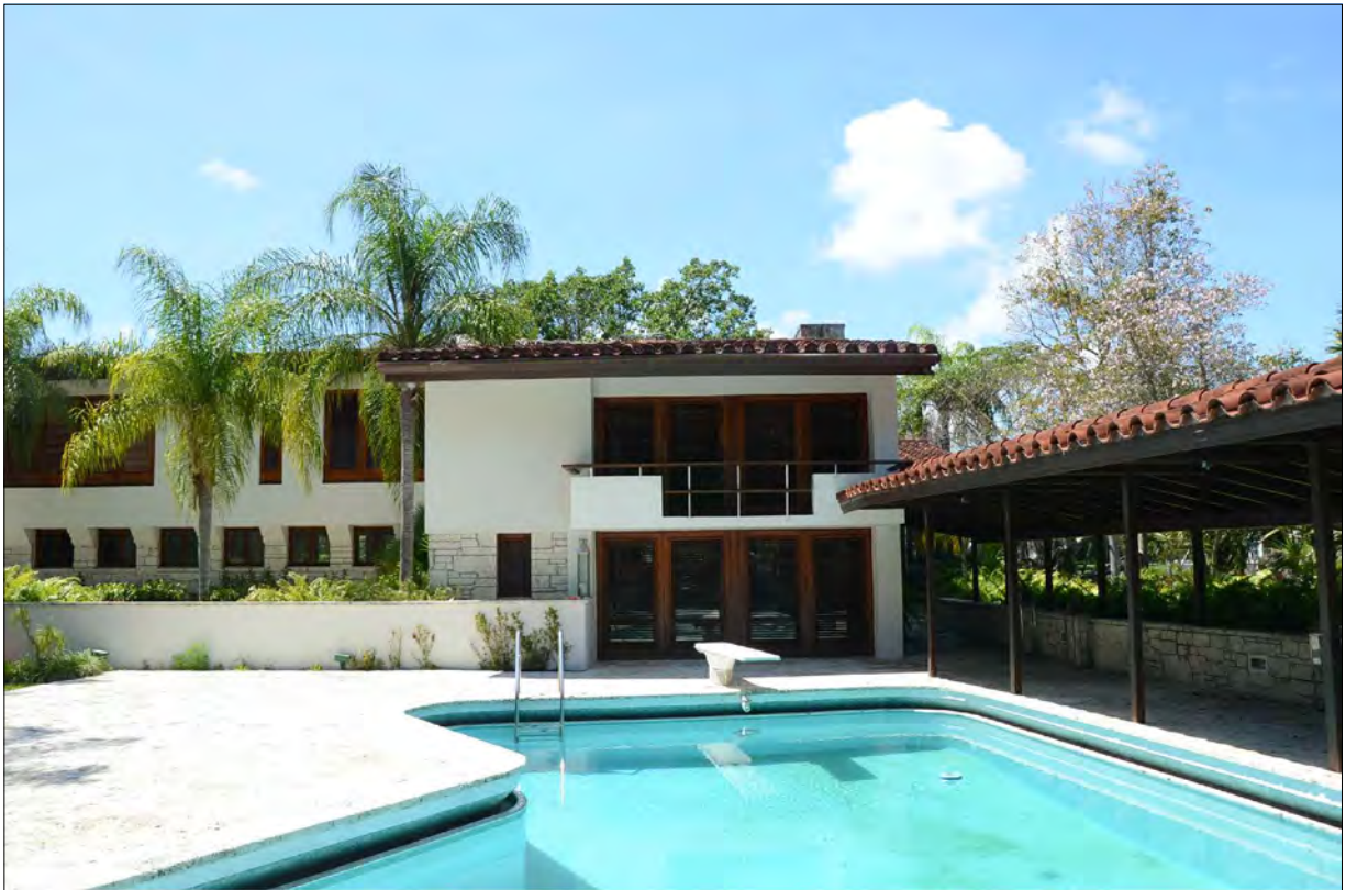
EXISTING RESIDENCE AND POOL AREA (ORIGINAL PARKER)
