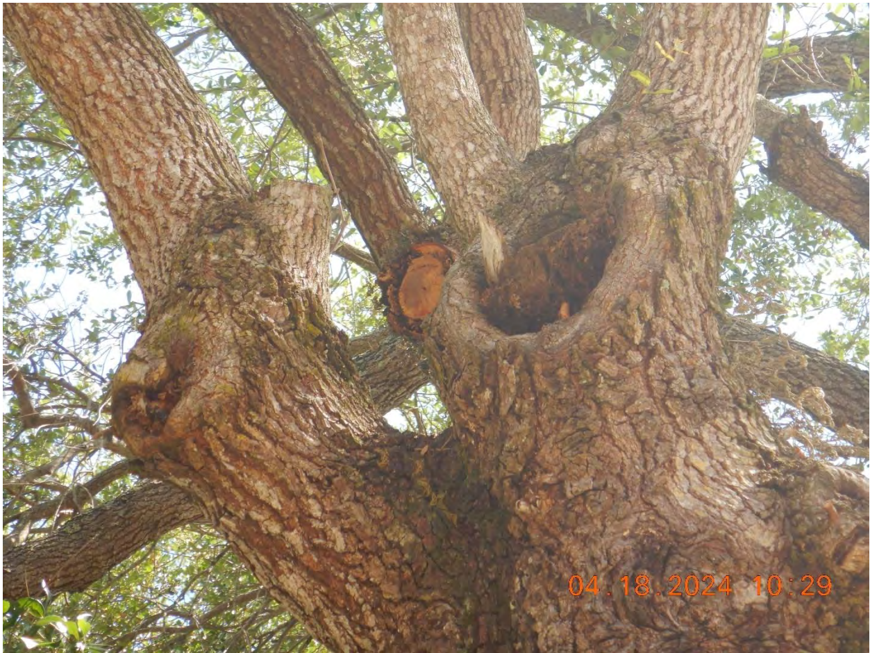
Decay where branches were removed.
