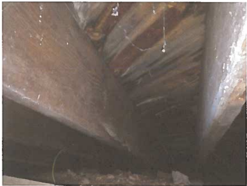
8 FIRST FLOOR FRAMING (EAST SIDE)
