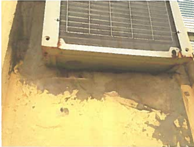
5. AIR CONDITIONING INSTALLATION
