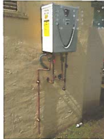
6. PENETRATION OPENINGS @ WH
