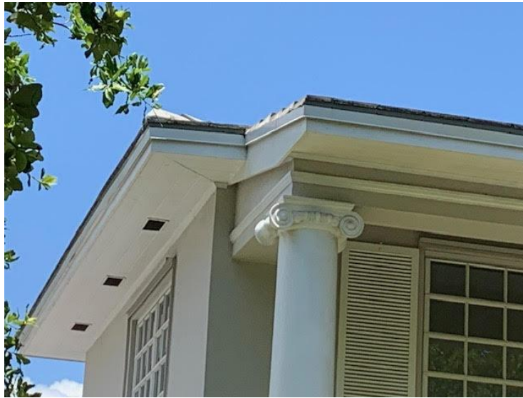
Closeup of capital under the overhanging eaves that surround the residence, Courtesy of HPACG
