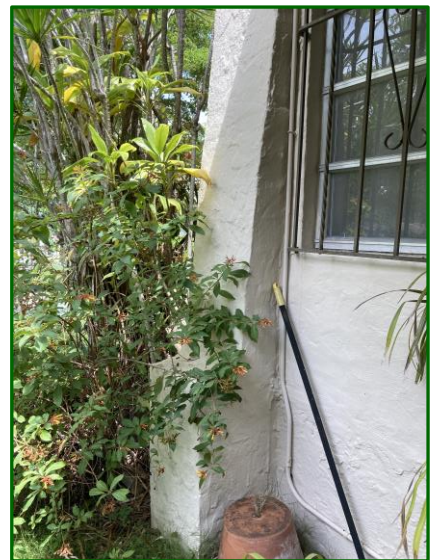
Figure 16: Southwest Corner, Looking West, 2023 Note: wing wall, differentiation of stucco indicating original entry porch window size
