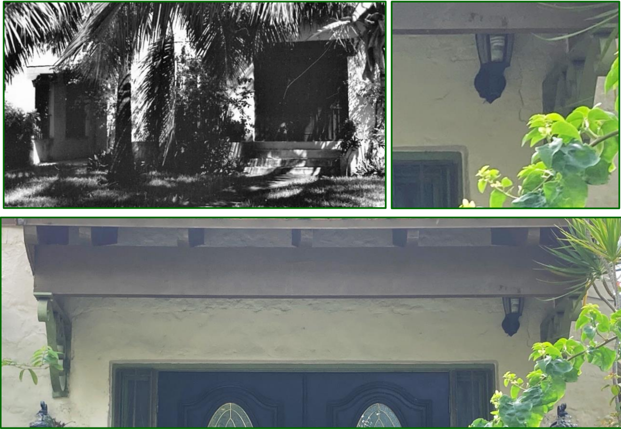
Figures 15: Front Entry Lintel Original Pecky Cypress Lintel, c.1940 [top left] Lintel with Stucco Cladding, Outline Discernable, 2023 [top right, bottom]
