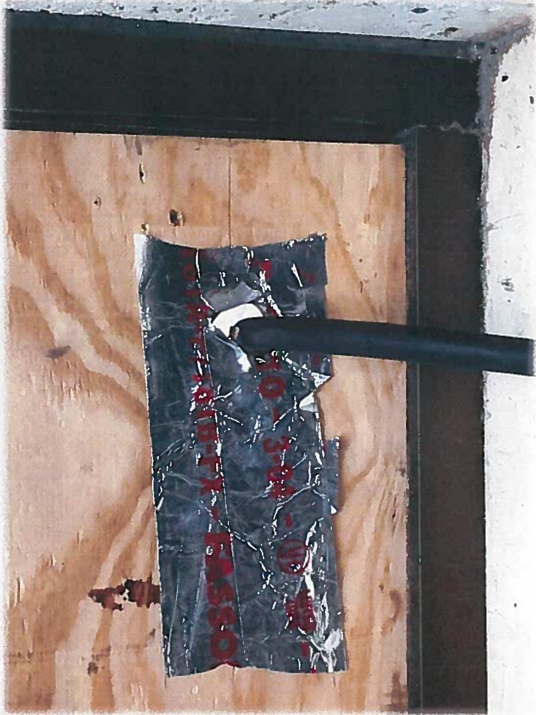
Plywood on window enabling portable air conditioner
