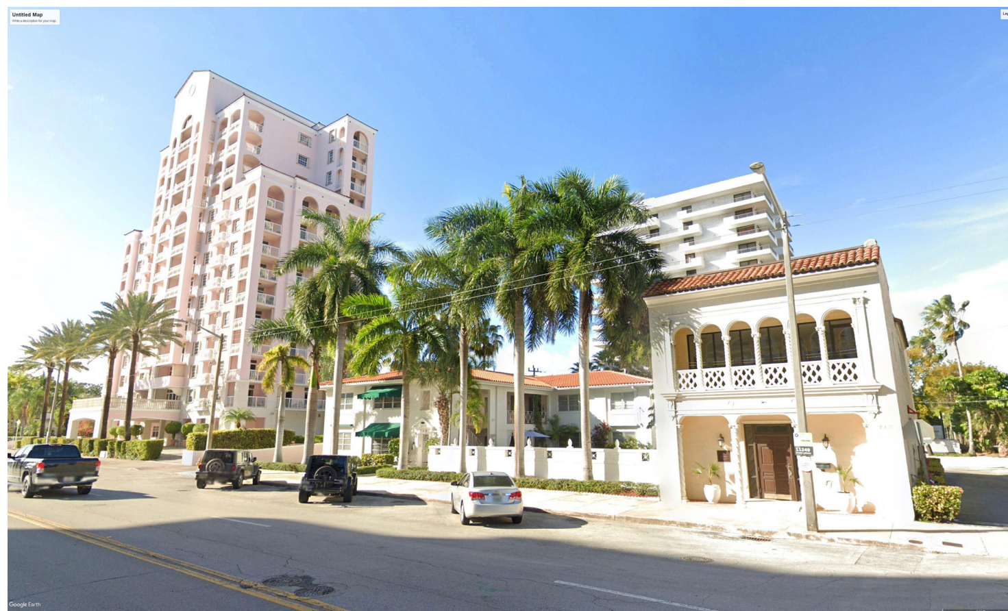
VIEW FROM SOUTH LOOKING NORTH
