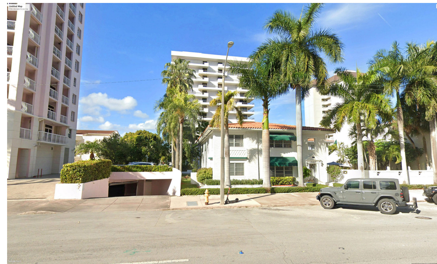
VIEW FROM SOUTH LOOKING NORTH
