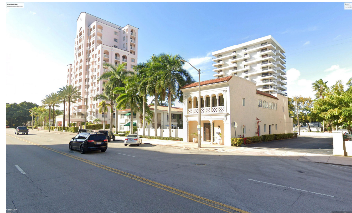
VIEW FROM EAST LOOKING WEST
