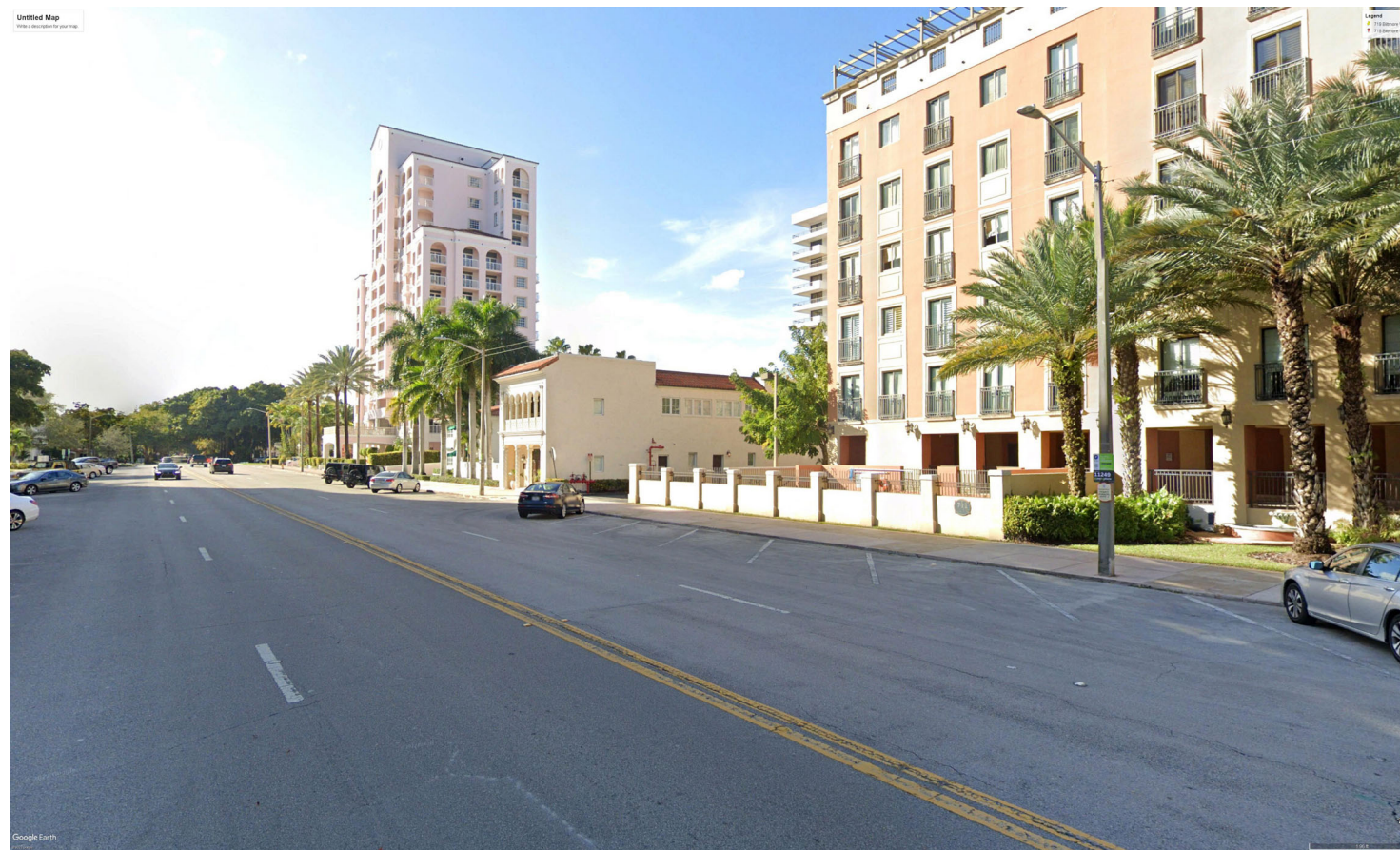
VIEW FROM EAST LOOKING WEST
