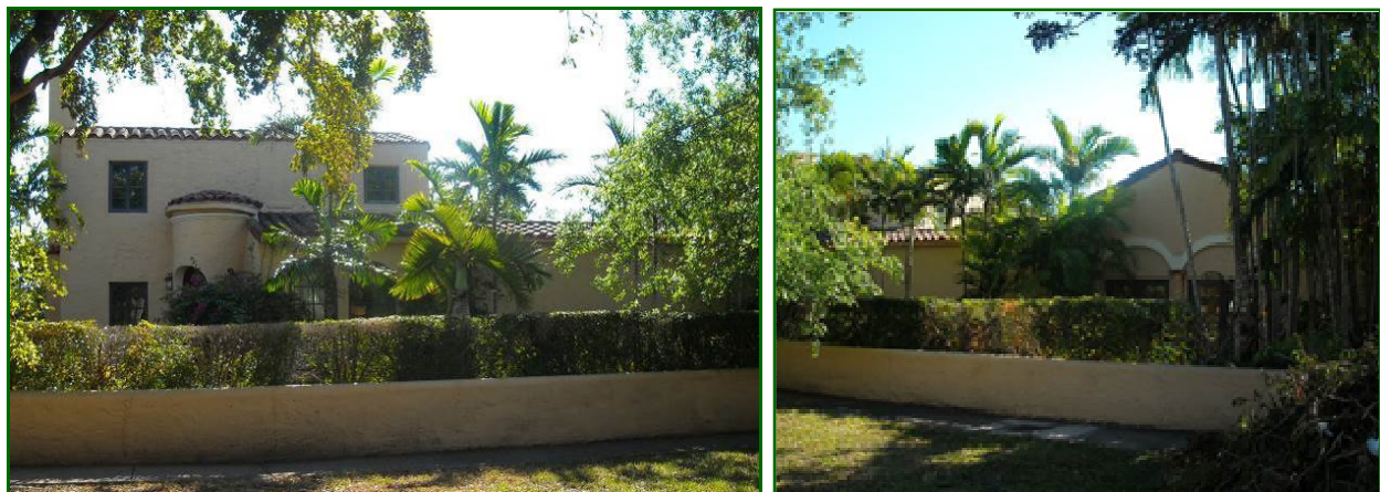
Figures 10: Front (west) Facade, 2018: Northern section (1925) [left]; Southern section (1982) [right]
