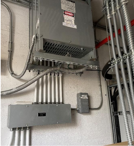
Figure 43: Types of wiring methods - PVC & MC
