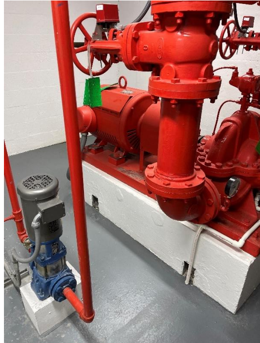
Figure 57: Fire Pump
