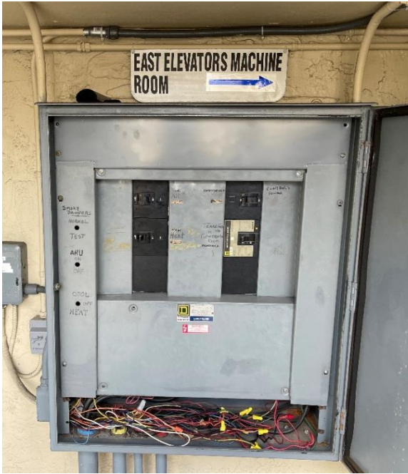
Figure 27: Roof Panel W
