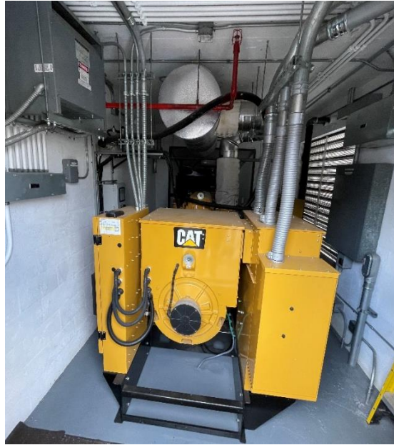
Figure 24: Emergency Generator
