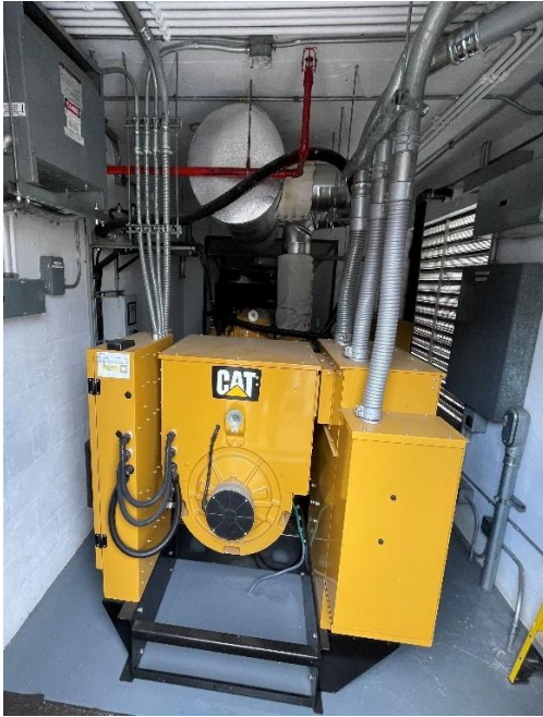
Figure 50: Emergency Generator
