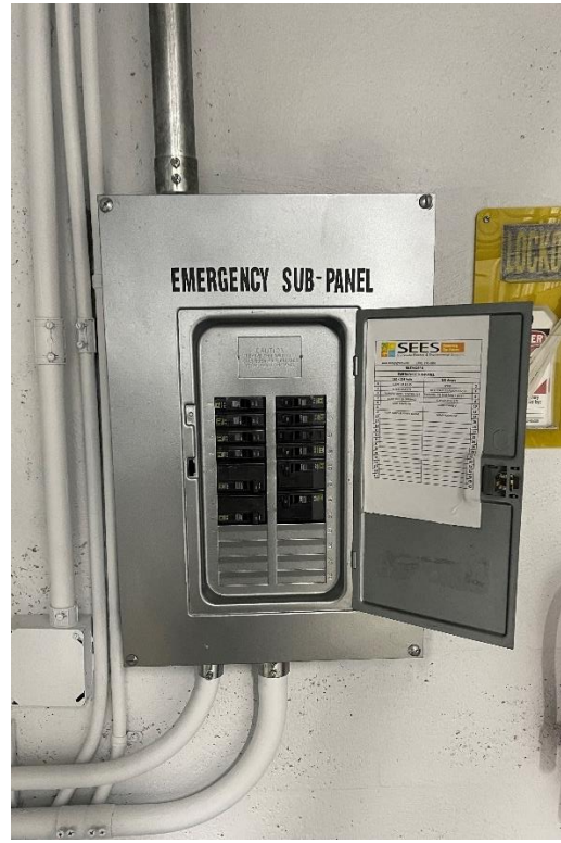
Figure 20: Emergency Sub-Panel
