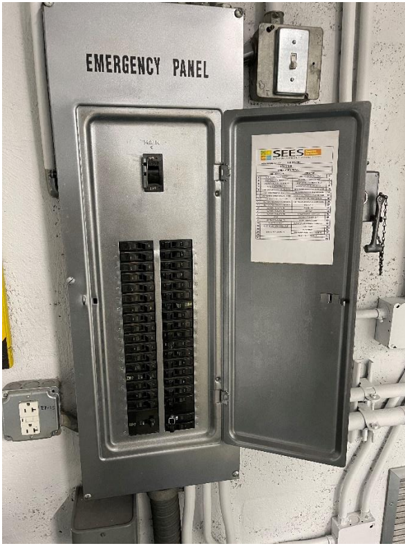
Figure 19: Emergency Panel
