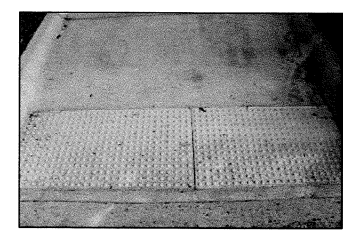
HANDICAP WARNING PAVEMENT-SEE CIVIL FOR DETAILS
