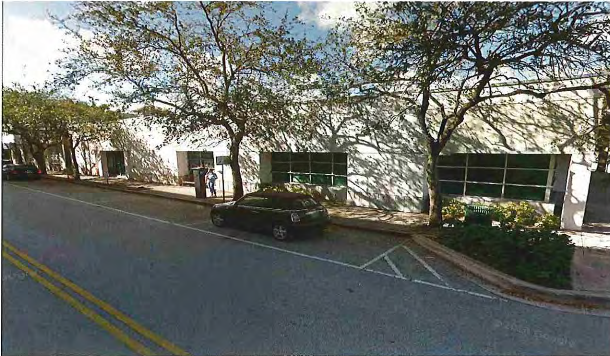
Property to the North End of Block on Laguna St
