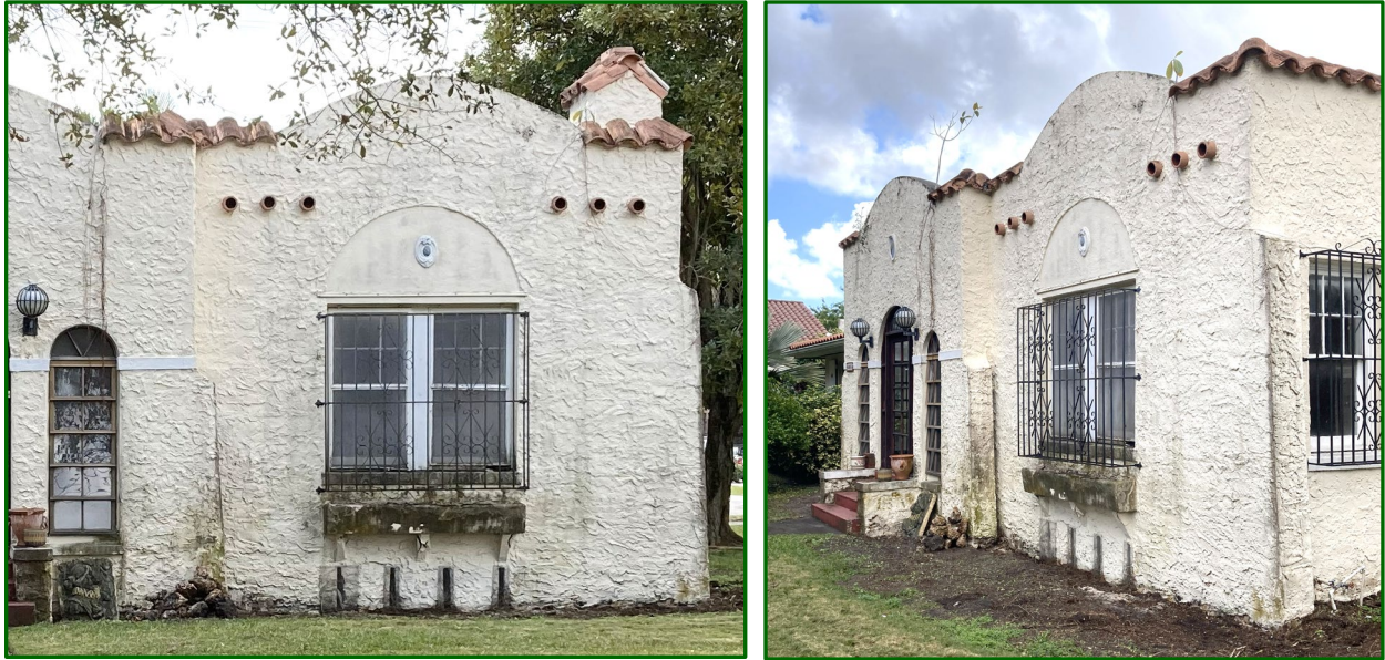
Figures 15: Front Façade, Western Bay, 2025
