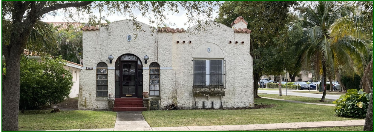
Figure 12: Front (North) Façade, 2025
