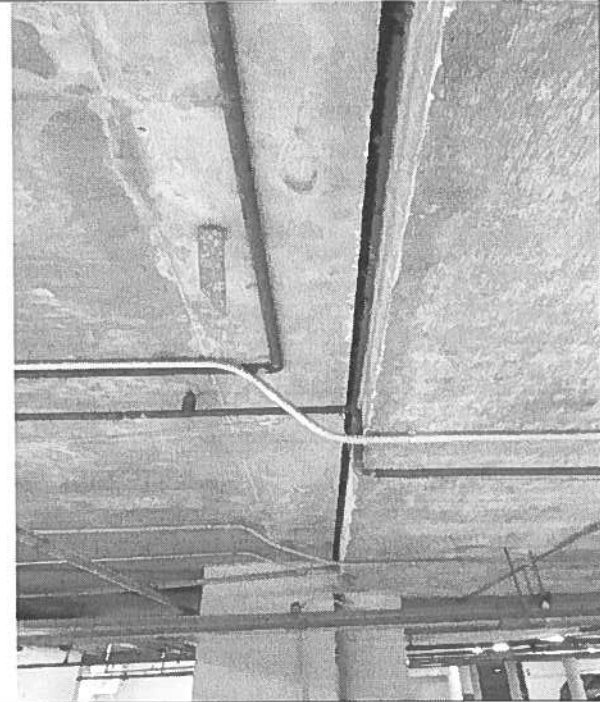
16. Expansion joint at garage
