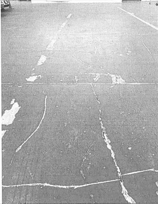
13. Non-structural cracks at topping upper garage
