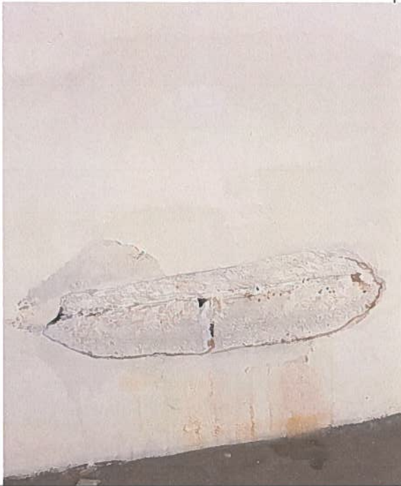
9. Concrete spalling at garage wall needs repair
