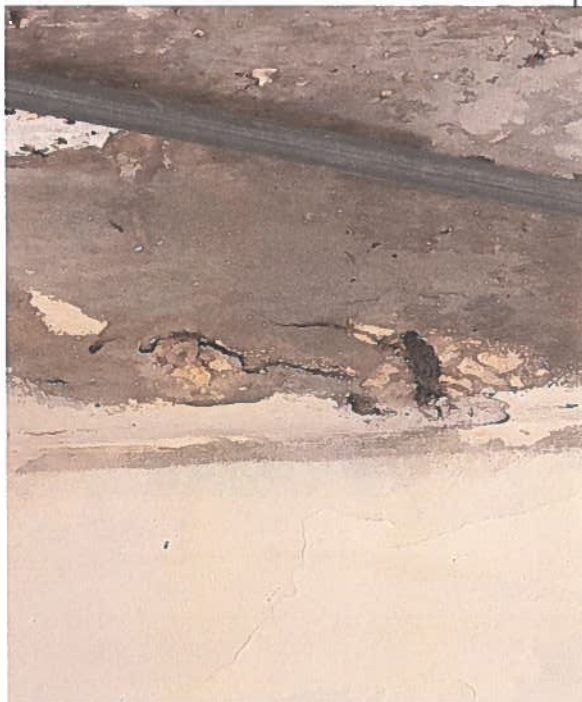
11. Concrete spalling at garage ceiling needs repair
