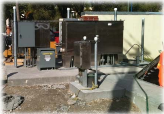
Project site during construction, December 2011
