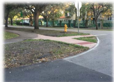
Recent sidewalk ADA improvement
