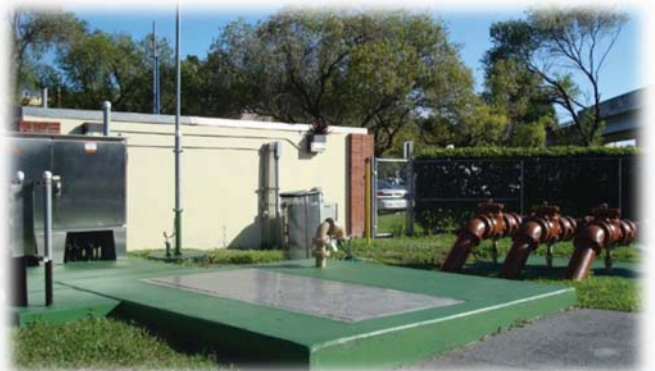
Project site after construction, February 2014
