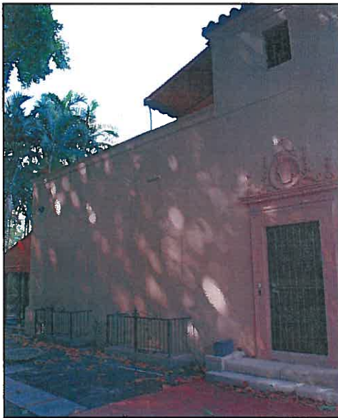
Figure 11: Front (South) Façade, 2017
