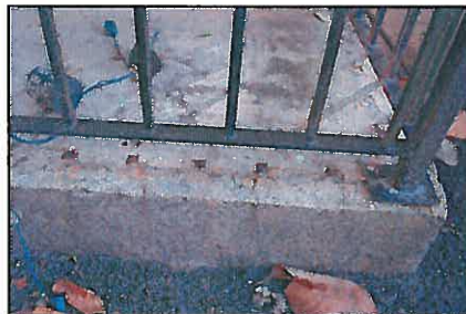
Figure 12: Wrought Iron Railing Detail, 2017
