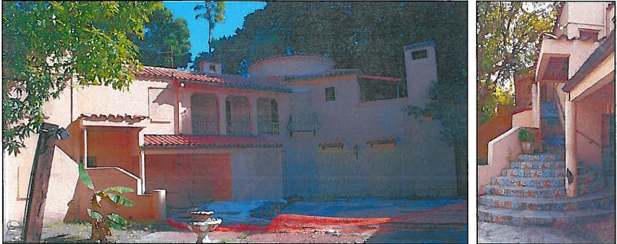
Figures 19 and 20: Rear (West) Façade, 2017 [left] and Stair Detail, 2016 [right]
