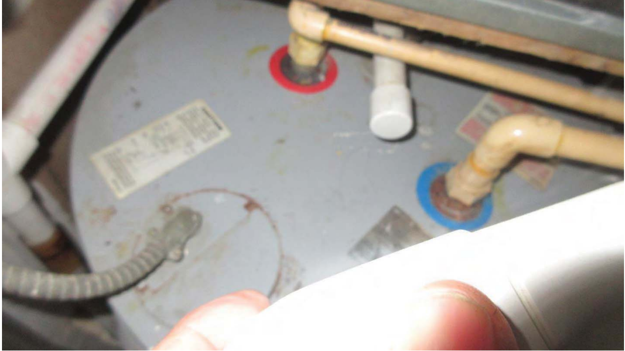
WIRING OF MECHANICAL EQUIPMENT.
