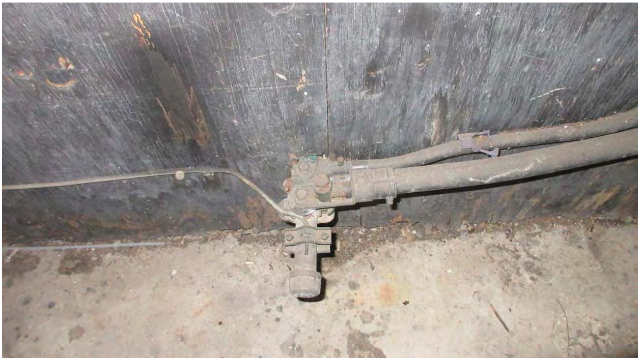
VIEW OF GROUNDING OF SERVICE.
