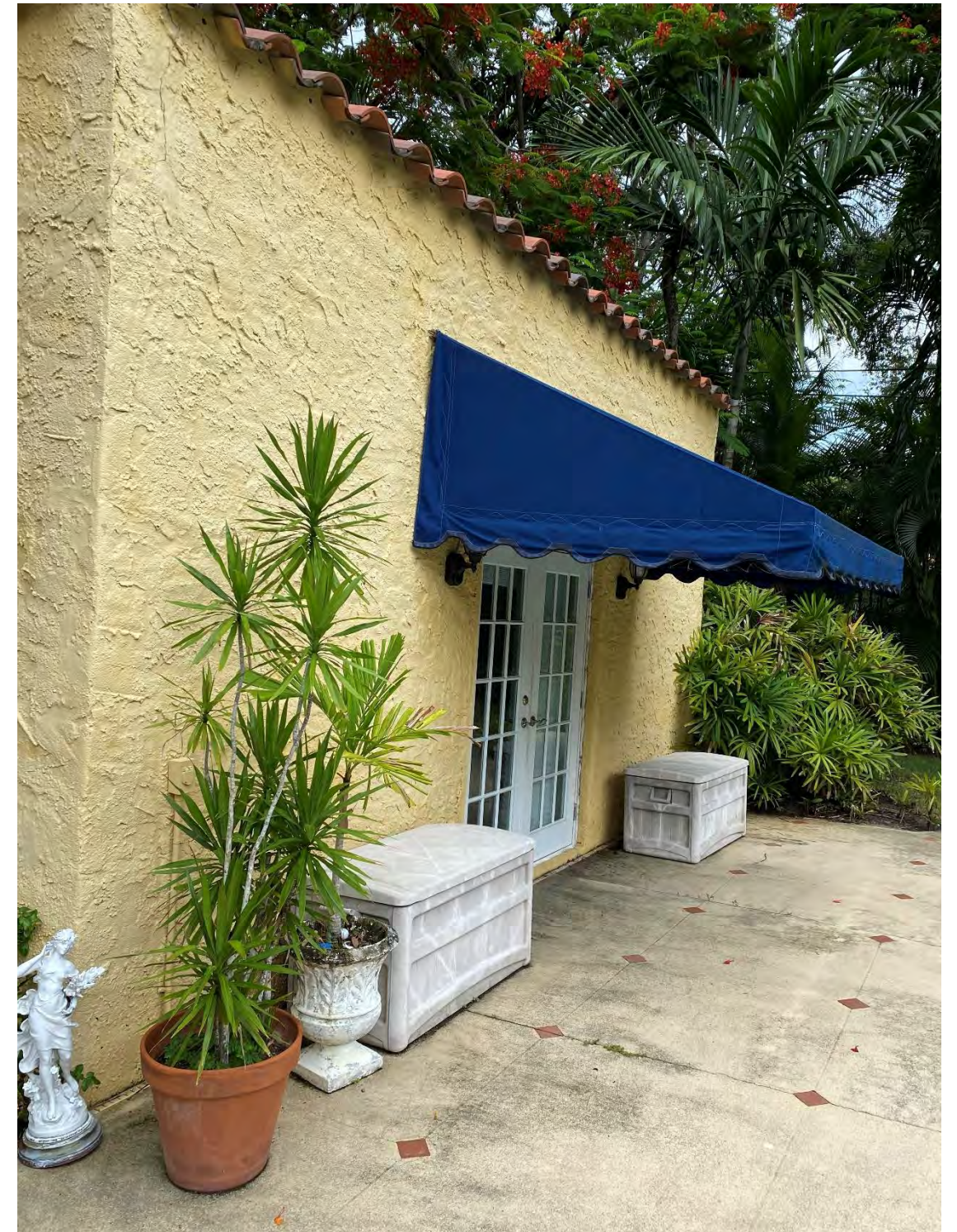
Accessory Building (East Façade)
