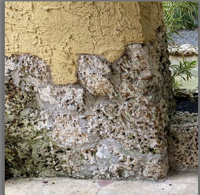
Rustic Coral Stone & Smooth Stucco Wall Finish (To Match Exist)
