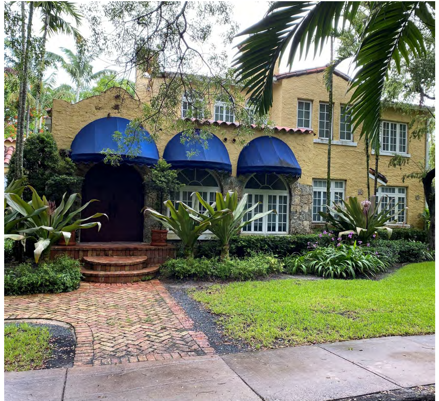
Front Elevation (Front Entry & Walkway)
