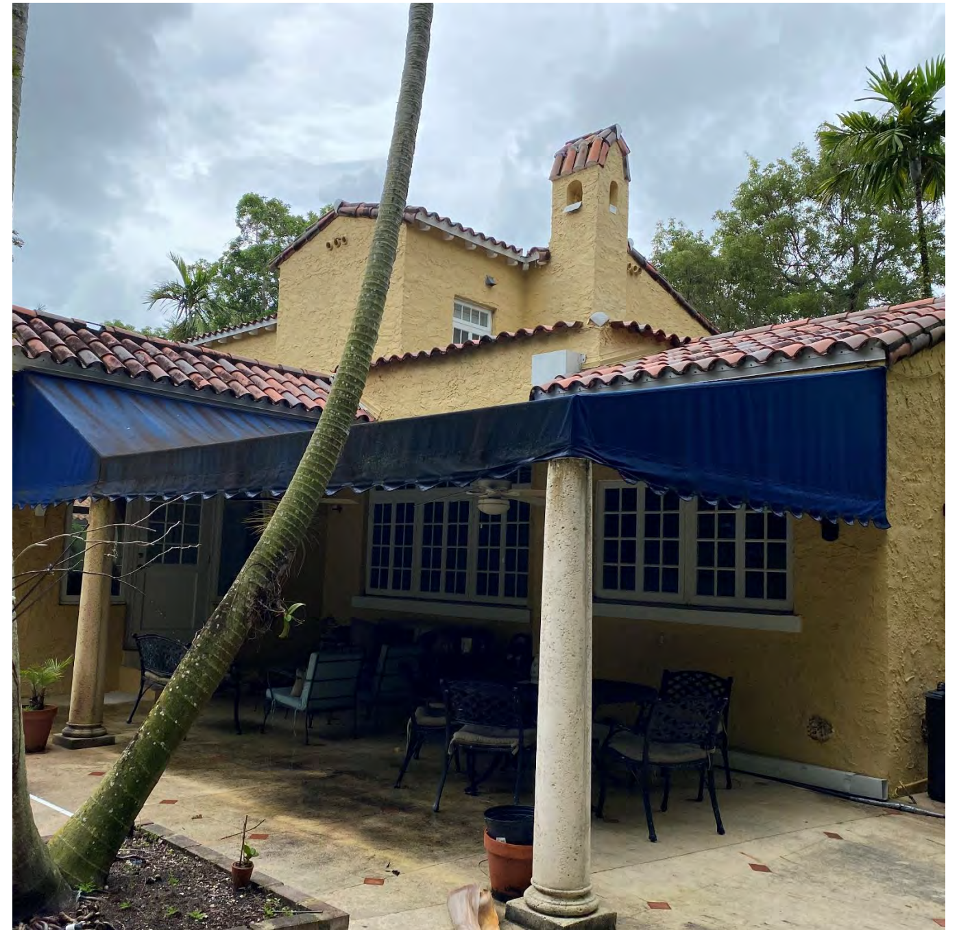
Rear Elevation (Main House & Terrace)
