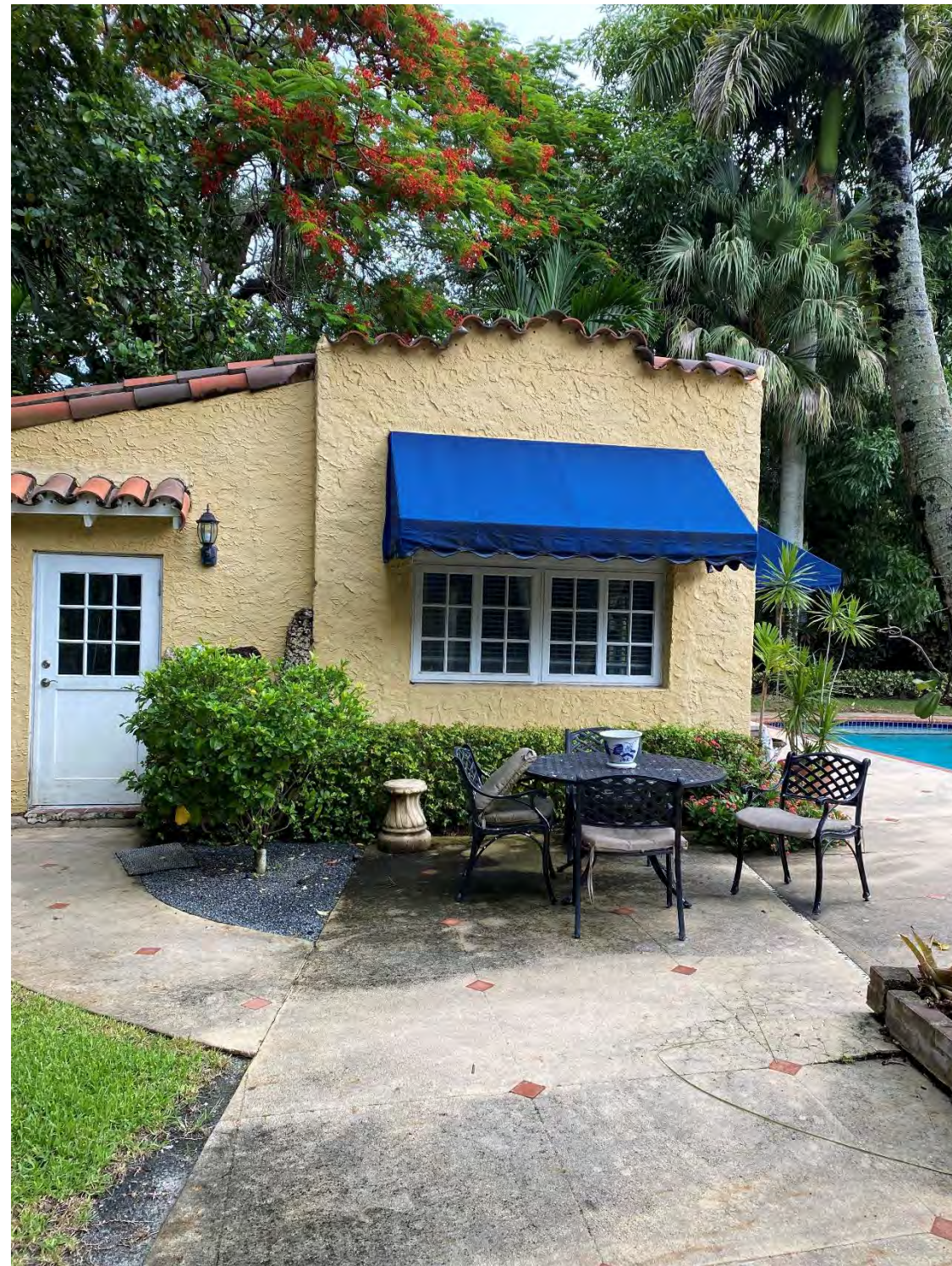
Accessory Building (North Façade/ Entrance)
