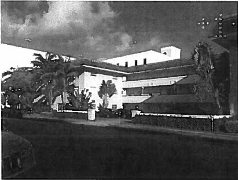
Photograph No. 1 (general building elevation)
