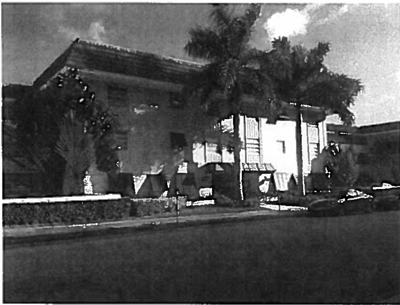
Photograph No. 2 (general building elevation)
