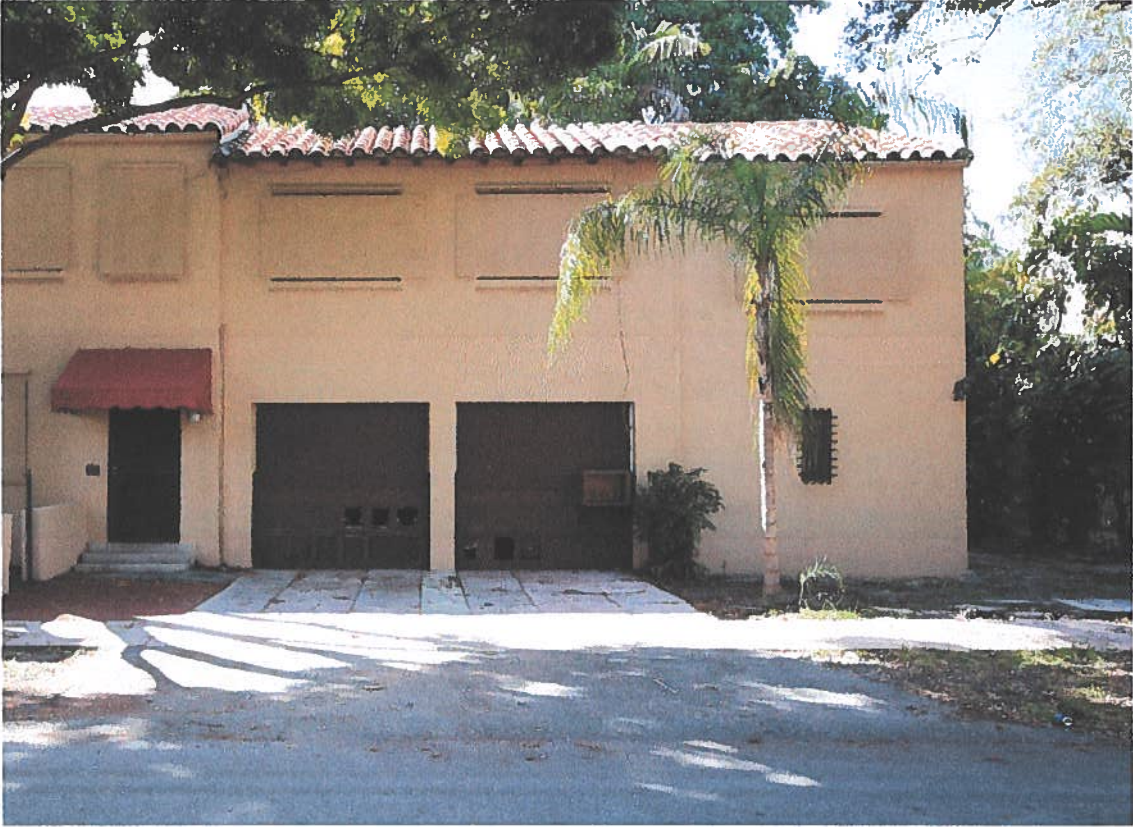
FEATURE 3: Driveway Photo Number: 17
