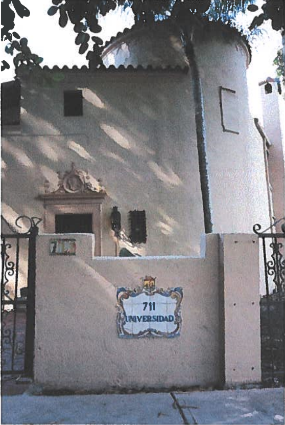
Elevation: South-East Existing Photo Number: 2
