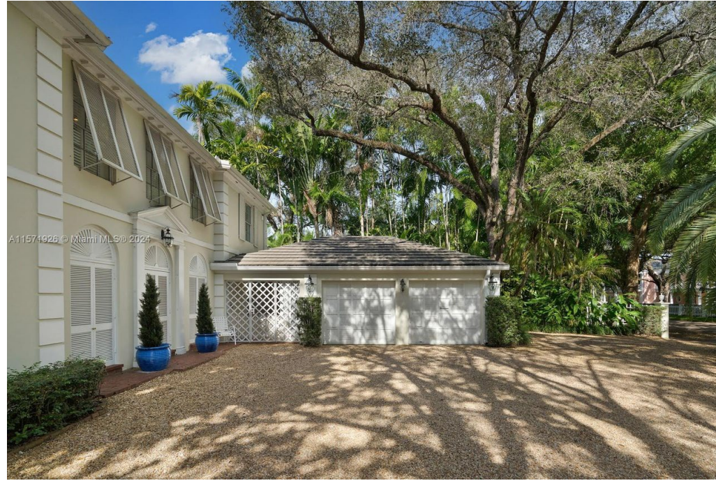
Existing House. Front view.
