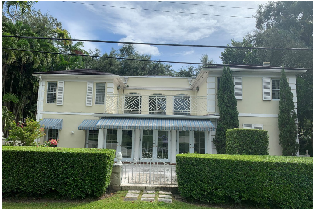
Existing house. Rear view
