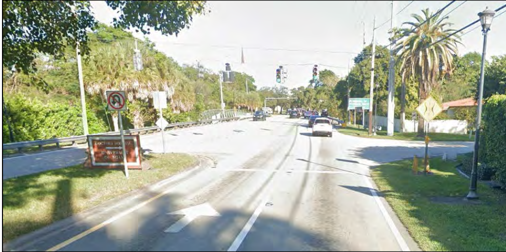
Photograph 3: View of Eastbound Approach at the Study Segment (One through lane and one shared through/right-turn lane)
