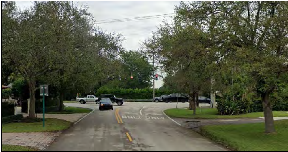
Photograph 2: View of Northbound Approach of the Study Intersection (One left-turn only lane and one right-turn only bay)
