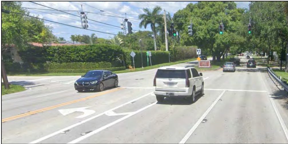
Photograph 4: View of Westbound Approach at the Study Segment (One left-turn bay and two through lanes)
