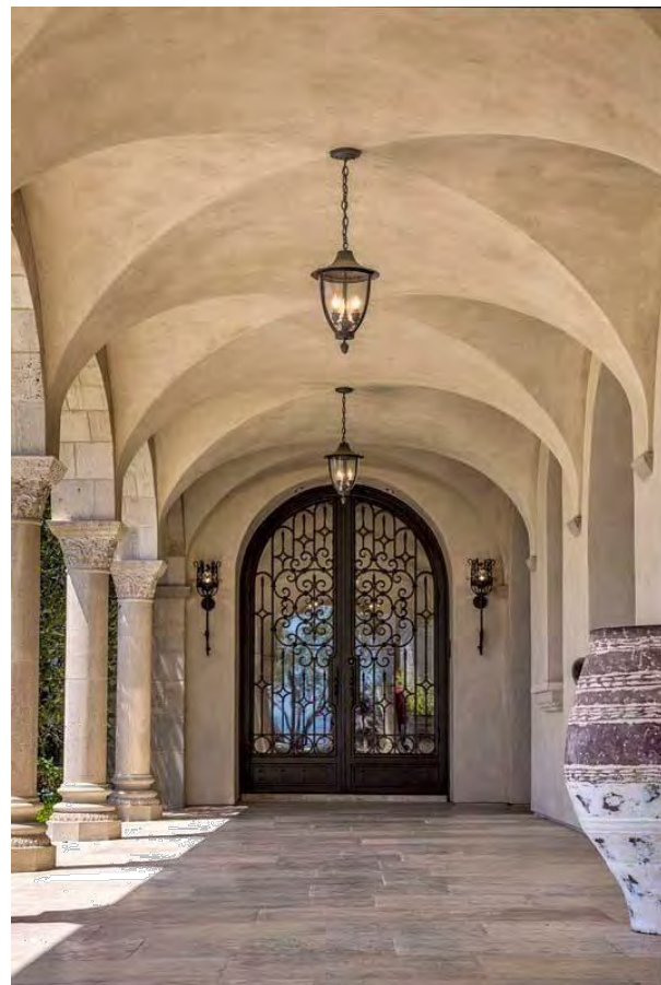
CLASSIC GROIN VAULT INSPIRATION
