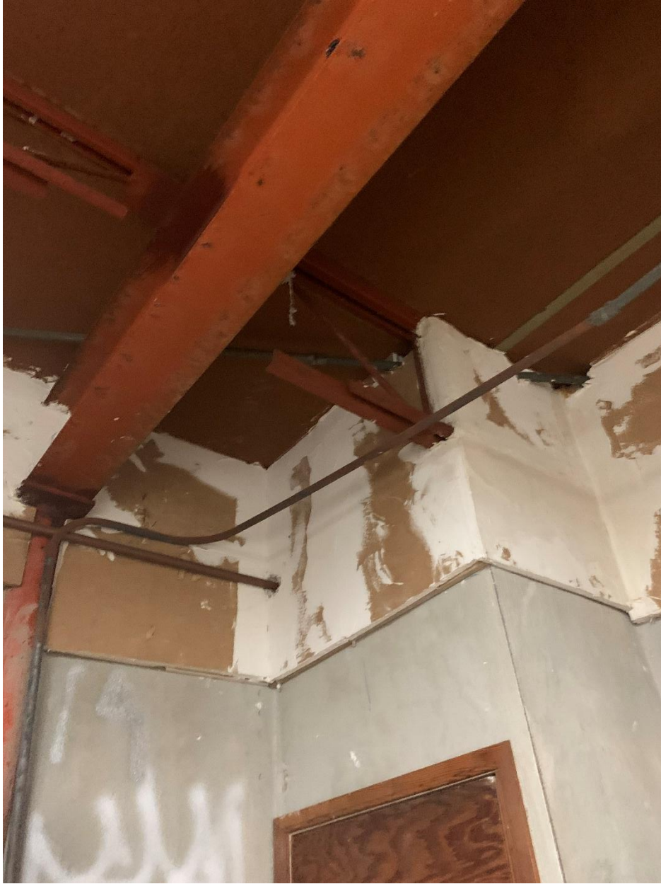
Structural Photo 7a1 (2) – 6915 S. Red Road – Roof Structure
