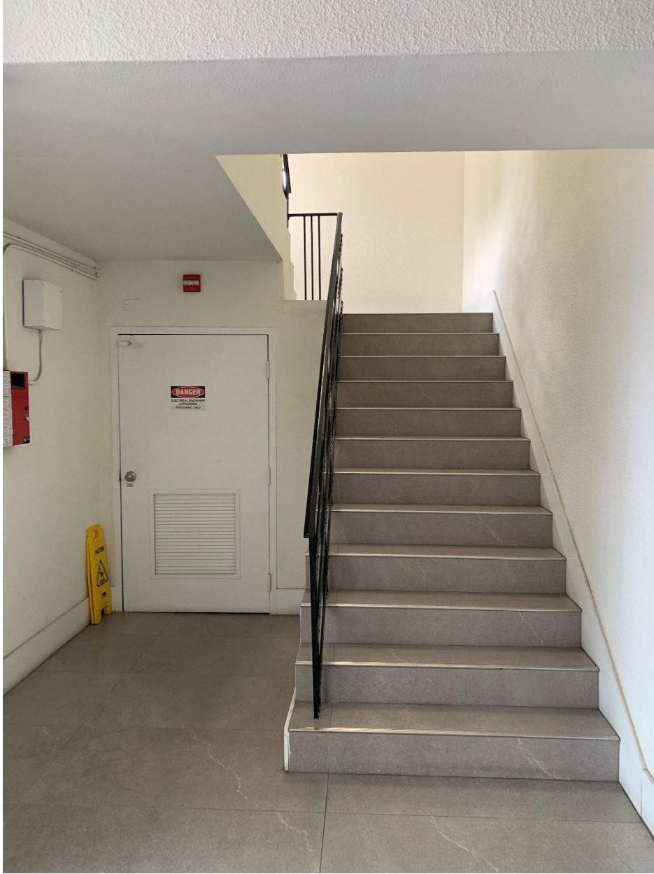
Structural Photo 7b3 – 6915 S. Red Road – Stairway
