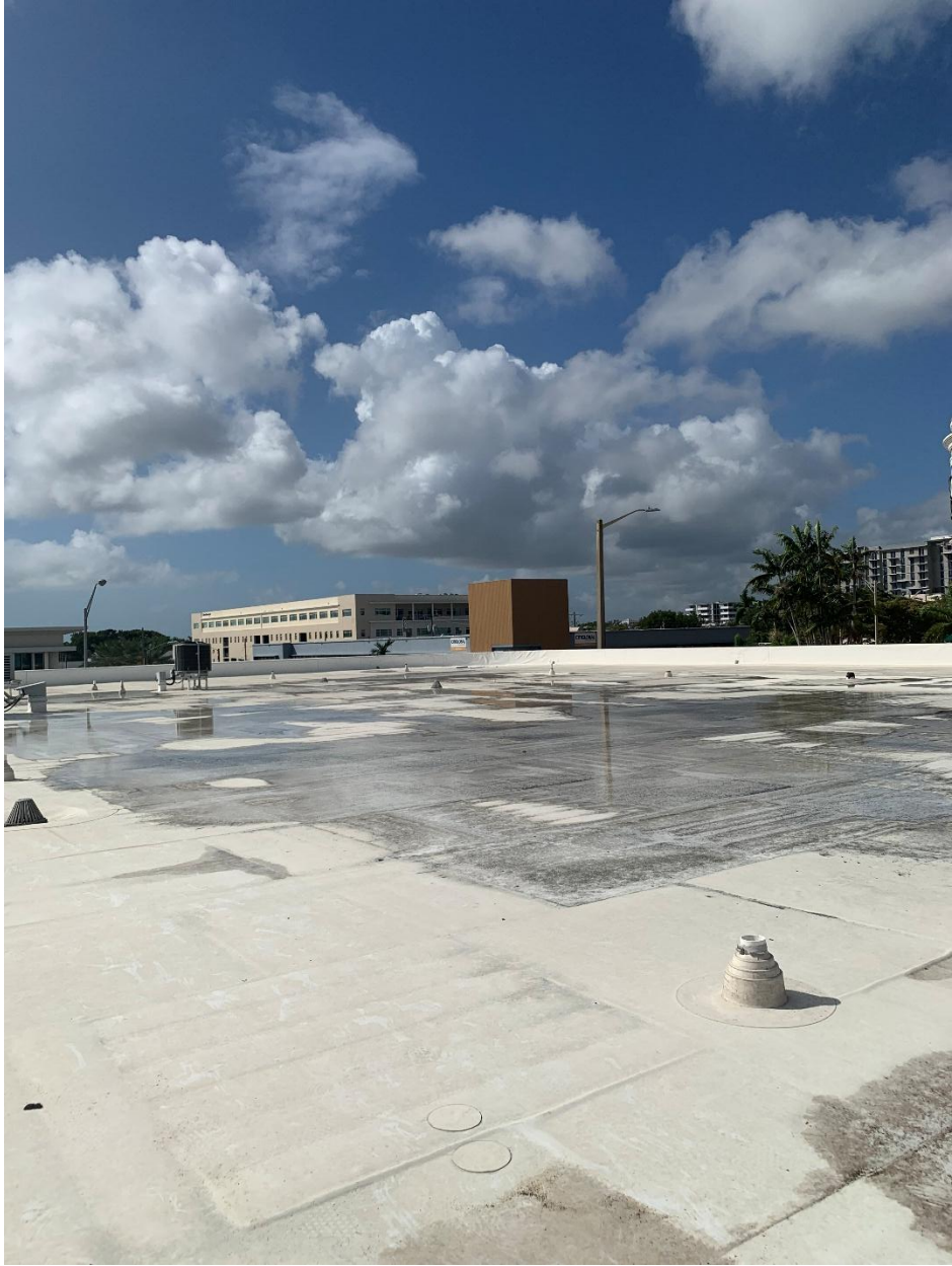
Structural Photo 7a6 – 6915 S. Red Road – Roofing
