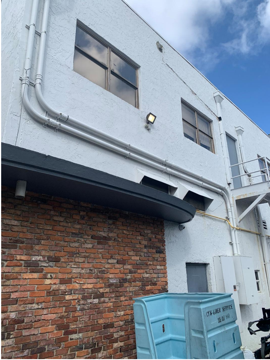
Structural Photo 6f (2) – 6915 S. Red Road – Exterior Veneer Finishes
