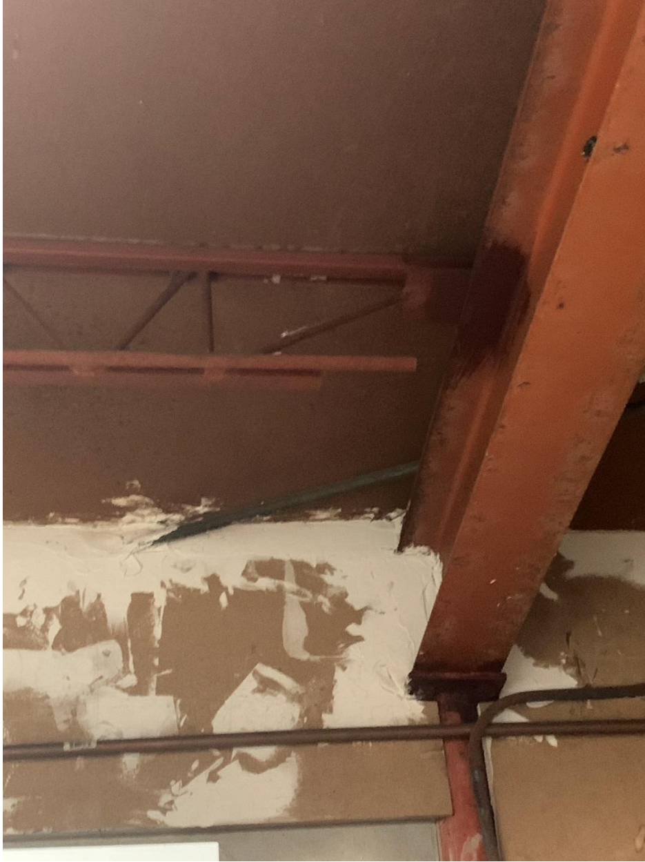
Structural Photo 8a, 8b, 8c – 6915 S. Red Road – Steel Framing
