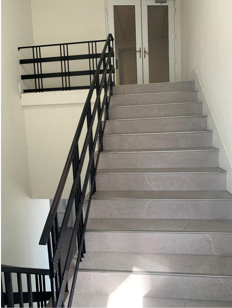
Structural Photo 7b5 – 6915 S. Red Road – Stairway and Handrails
