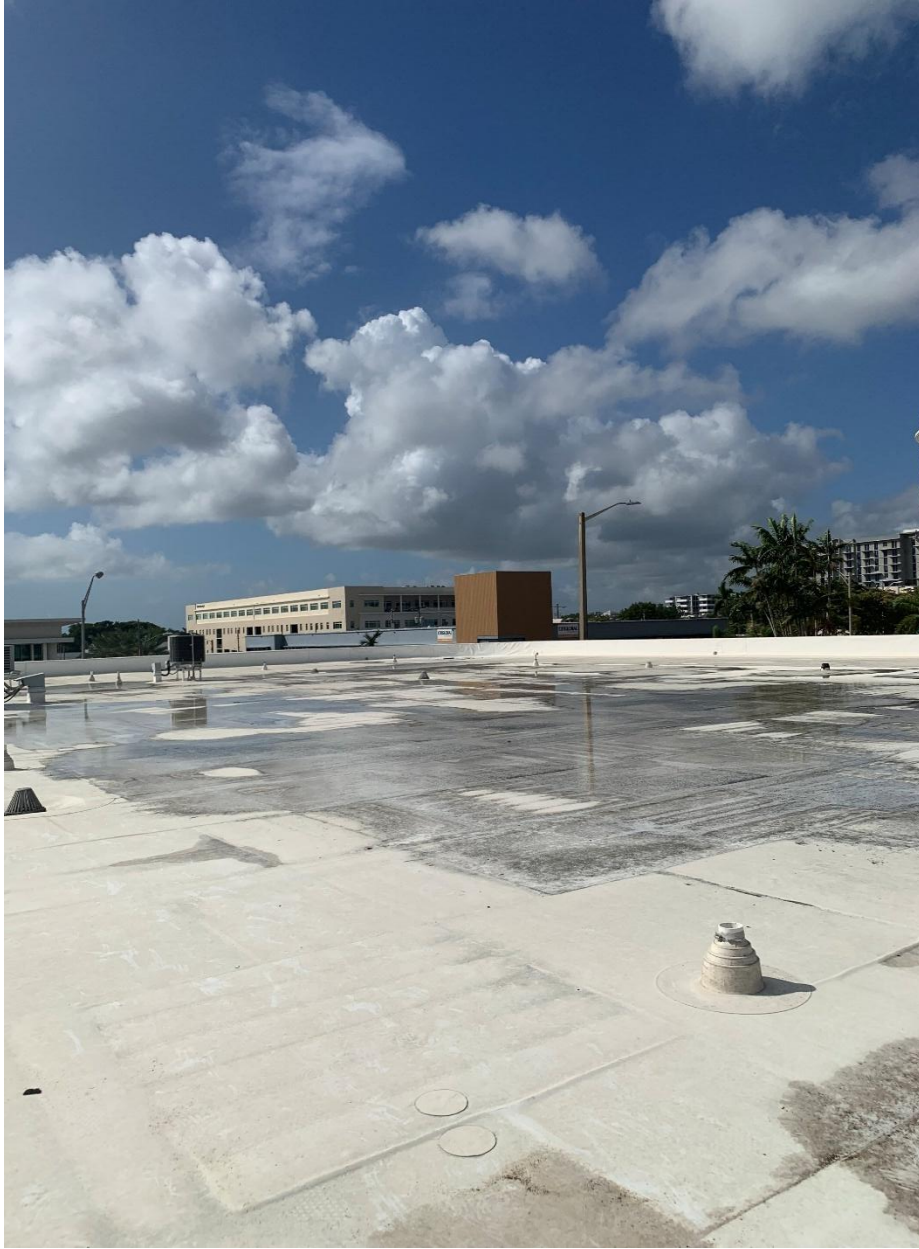
Structural Photo 7a1 (1) – 6915 S. Red Road – Roof Covering
