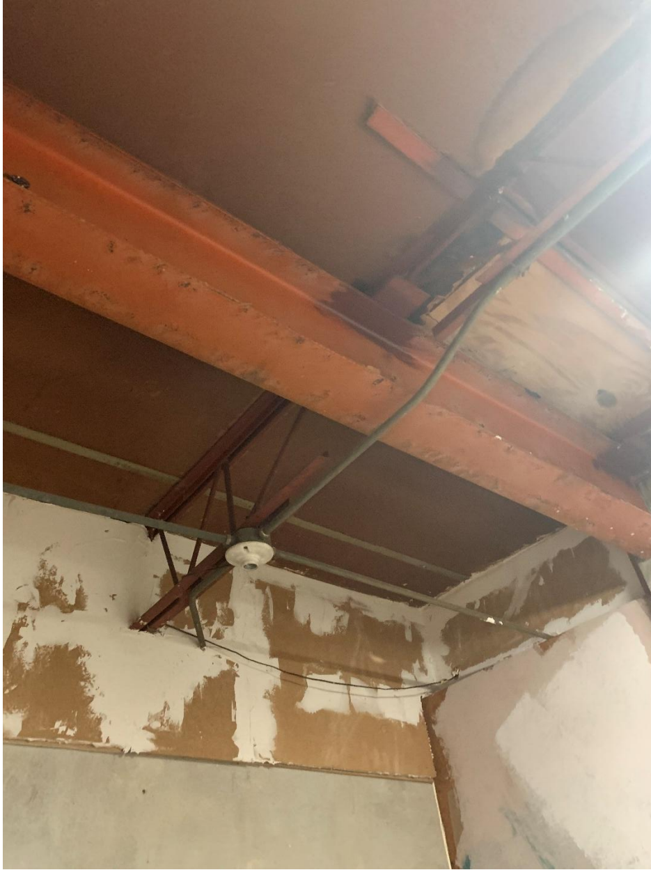
Structural Photo 7b1 – 6915 S. Red Road – Floor Structure
