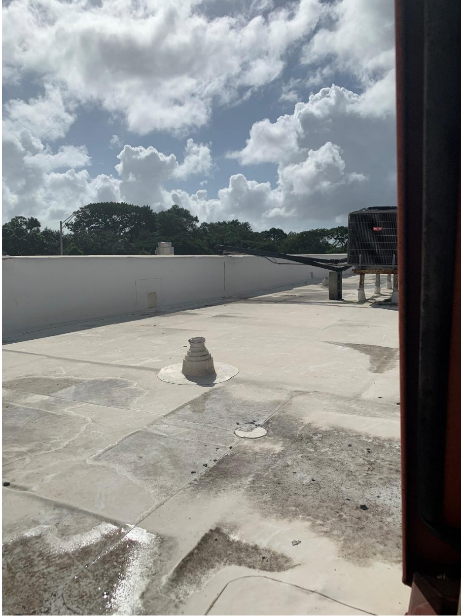
Structural Photo 7a3 (2) – 6915 S. Red Road – Roof Scuppers
