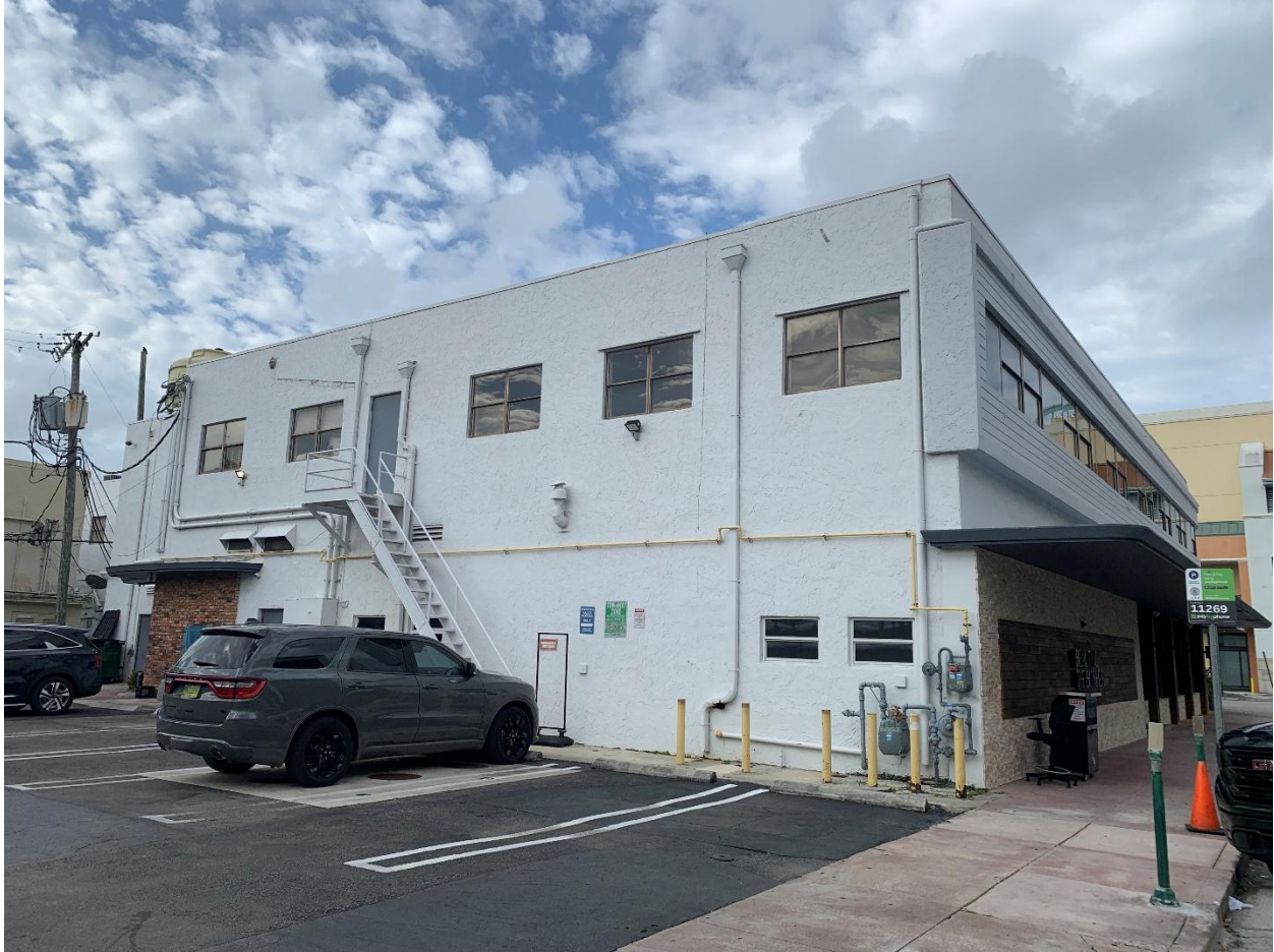
Structural Photo 10 (1) – 6915 S. Red Road – Windows and Storefronts
