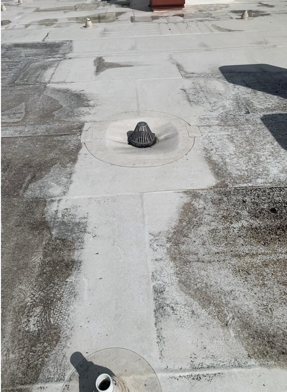
Structural Photo 7a3 (1) – 6915 S. Red Road – Roof Drains
