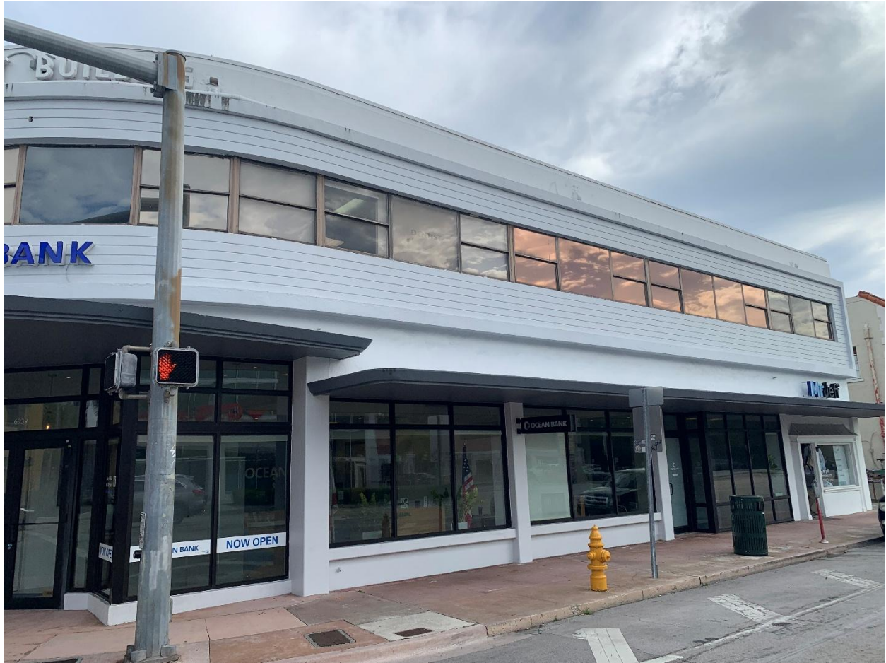
Structural Photo 5c – 6915 S. Red Road – General Condition of Finishes
