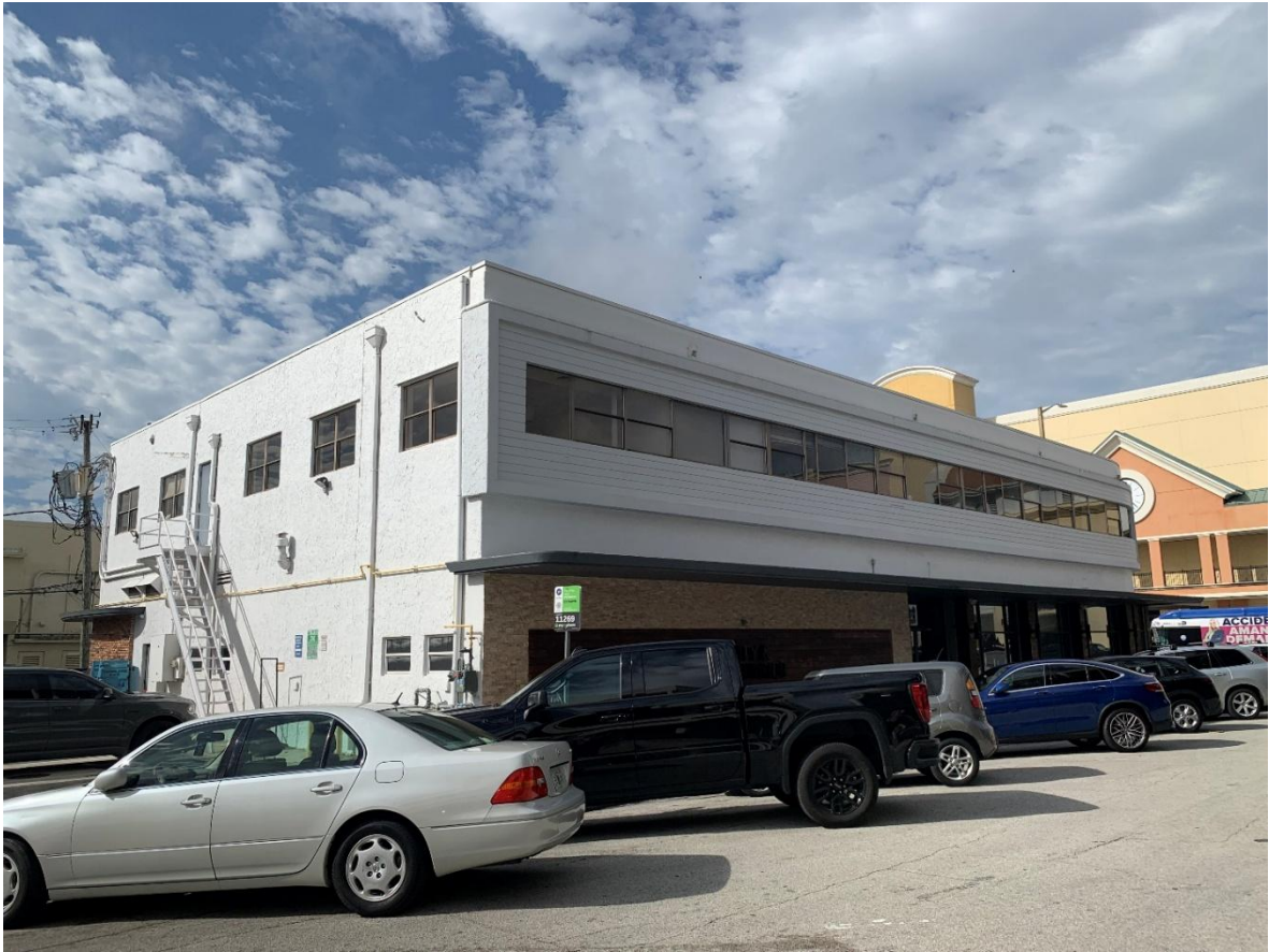
Structural Photo 5a – 6915 S. Red Road – Present Condition of Overall Structure
