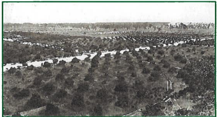
Figure 1: Streets in Coral Gables Under Construction, July 22, 1922
