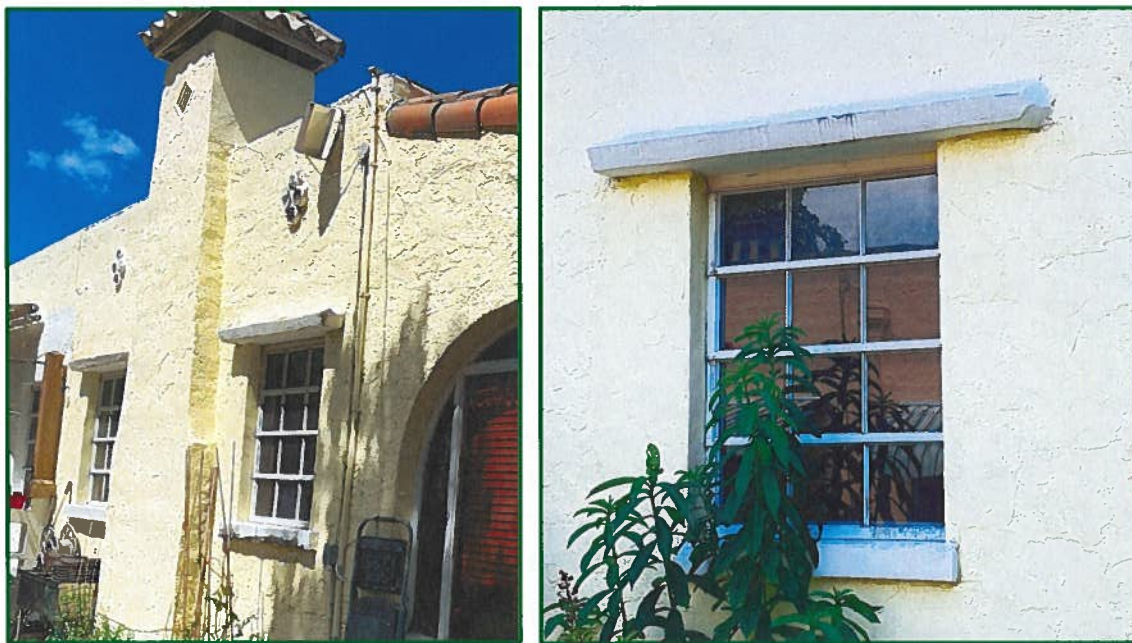
Figures 25: Flared Hoods Feature Over Windows, 2022 West Façade [left]; Lintel Detail, East Façade [right]
