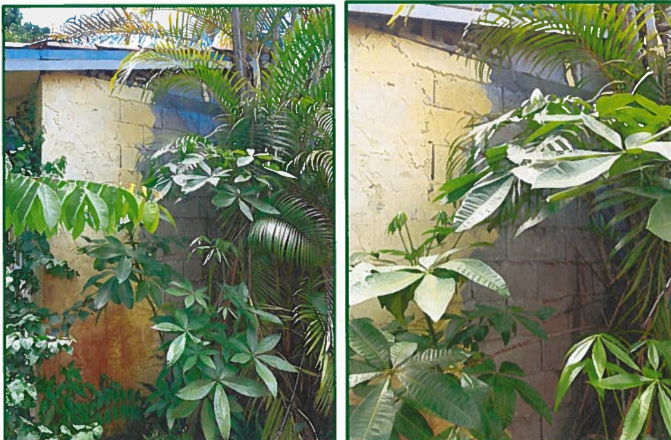
Figures 22: East Façade of c. 2011 Addition: Southeast Corner of Home, 2022
