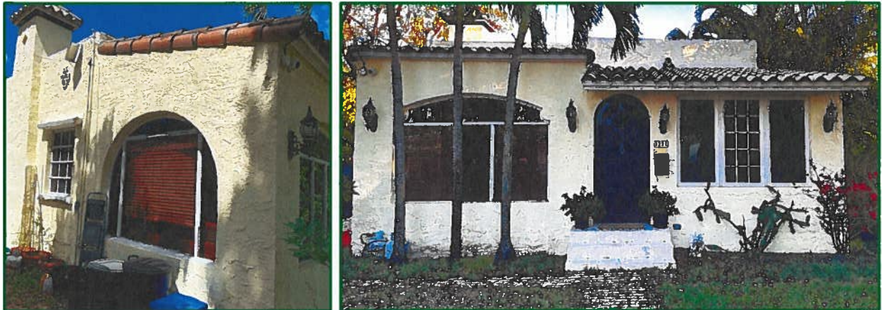
Figures 21: Front (South) Façade [right] Courtesy of Owner Note: porch enclosure extends beyond the east façade of the original home Southwest Corner, Arched Opening of Original Screened Porch, 2022 [left]
