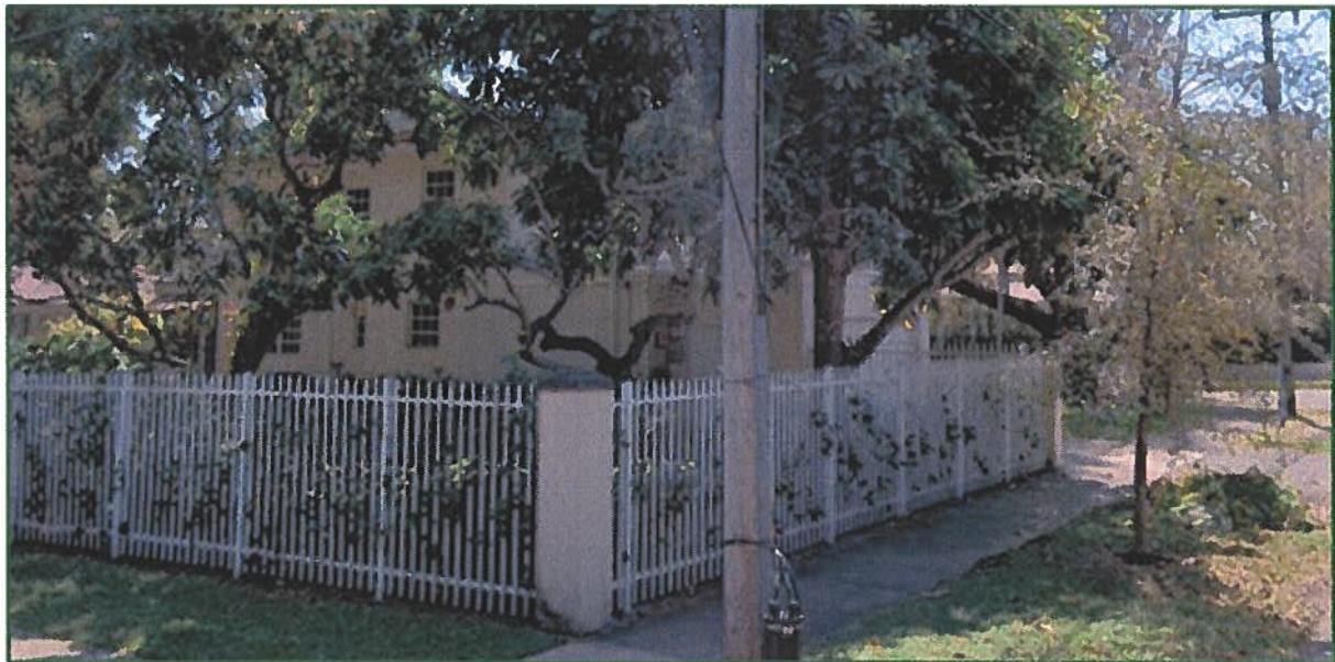
Figures 11: 649 Palmarito Court West Façade, Southwest Corner [top]; Northwest corner of Property [bottom] Courtesy of Google Earth
