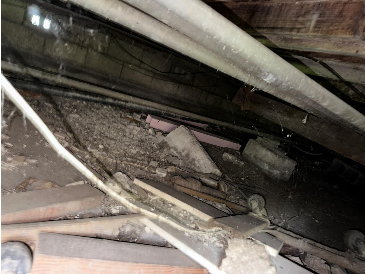
Wood joist on floor deck
