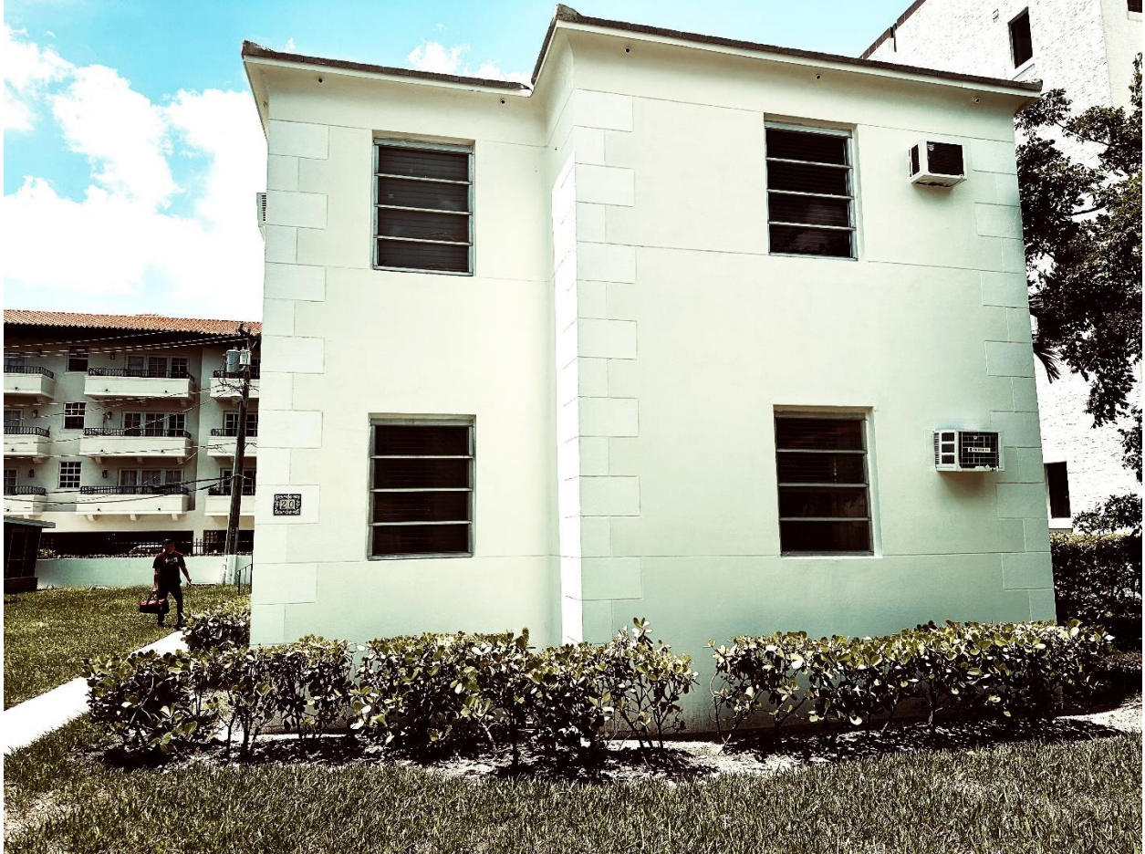
Front Elevation (NORTH) street view
