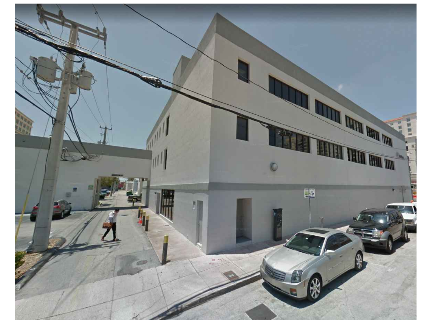
3. EXISTING BANK BUILDING - FROM GALIANO
