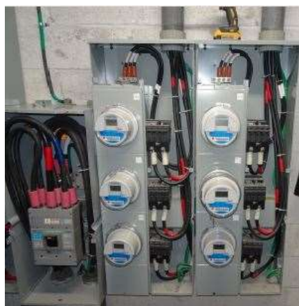
West Tower meter stack
