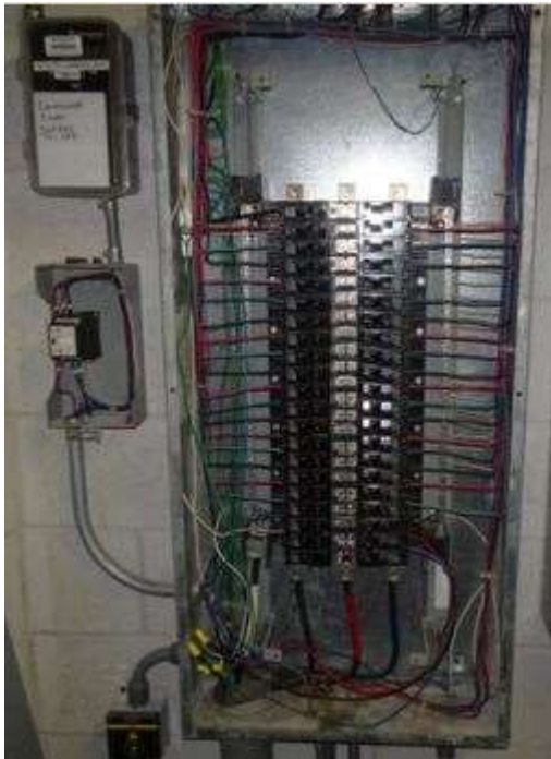
South Tower HA
