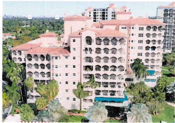
Photo-66: Photograph of South Elevation of South Tower.
