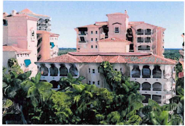
Photo-64: Photograph of West Elevation of West Tower.
