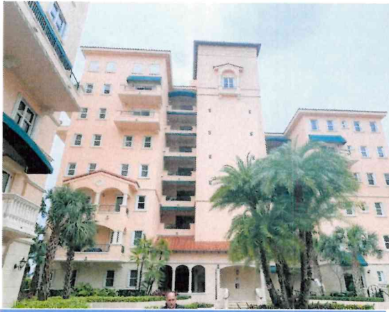
Photo-65: Photograph of North Elevation of South Tower.
