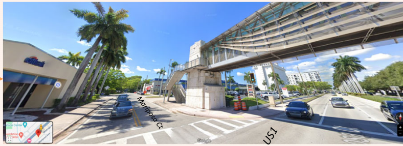
US1 & Mariposa Ct intersection (northeast)
